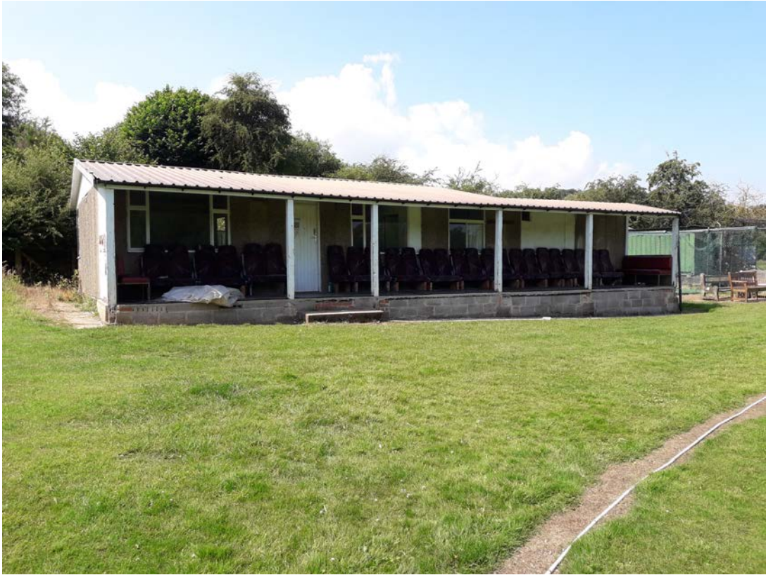
Photo showing existing pavilion.
