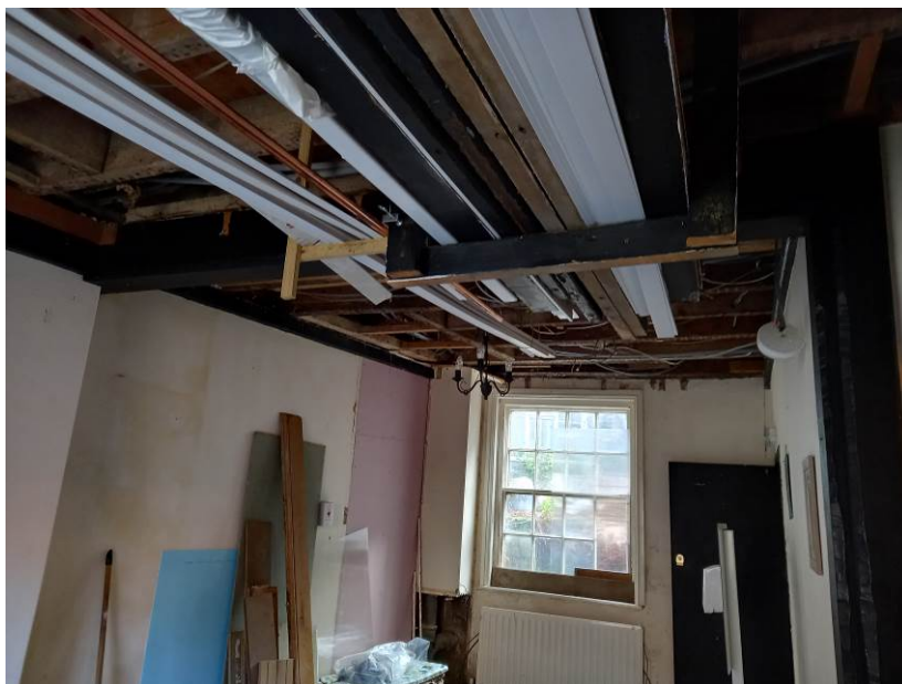
This photograph shows the 1 st floor internal space.
