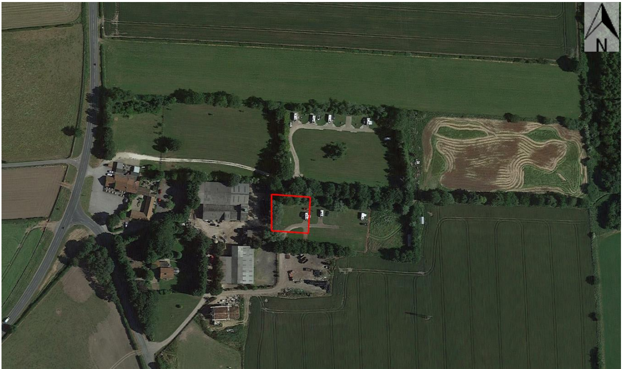
Figure 1. Approximate boundary of the proposed development outlined in red (aerial imagery dated 2018).
