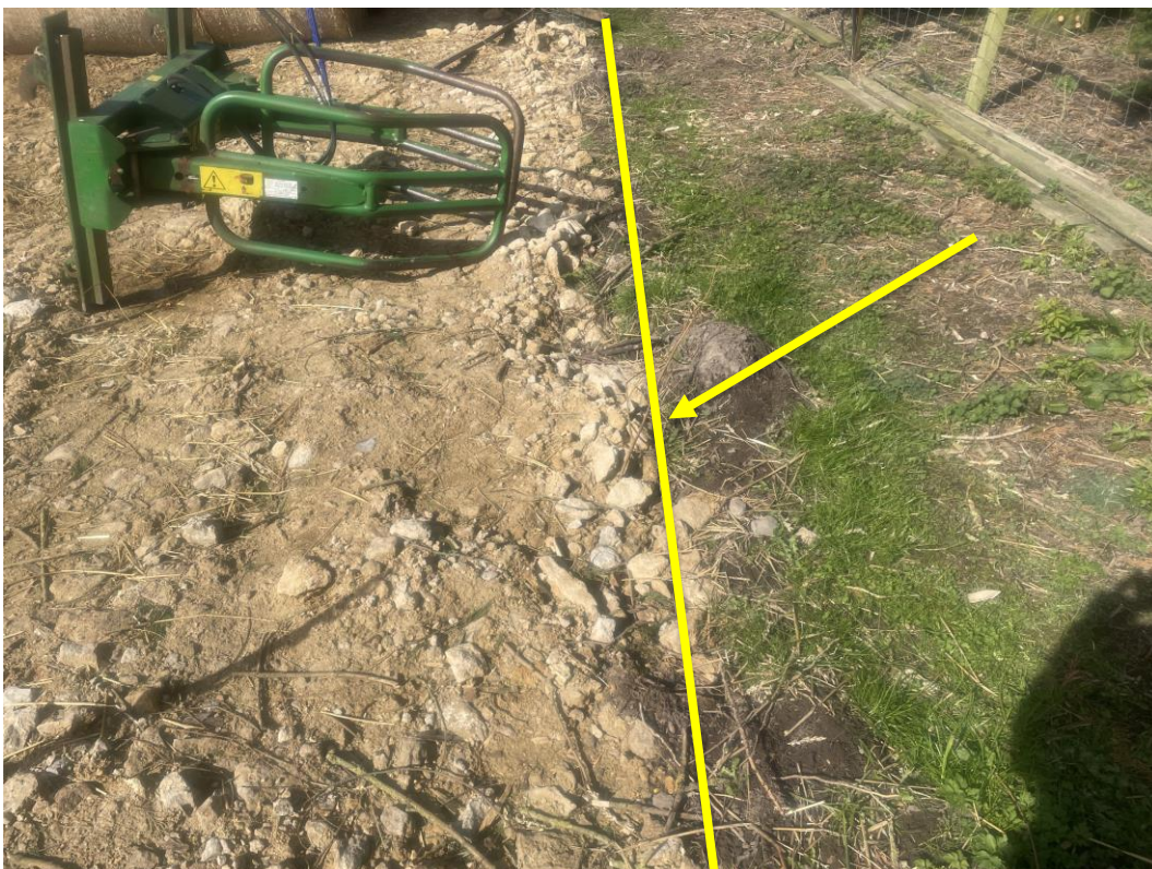
Image 8 – Depth of excavation is between 300-400 mm below the existing ground level, back fill with hardcore and subsequent compaction of the area will have removed the majority of rooting here.
