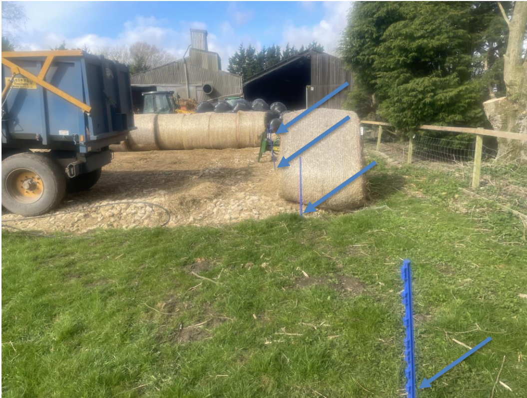
Image 8 – Depth of excavation is between 300-400 mm below the existing ground level, back fill with hardcore and subsequent compaction of the area will have removed the majority of rooting here.
