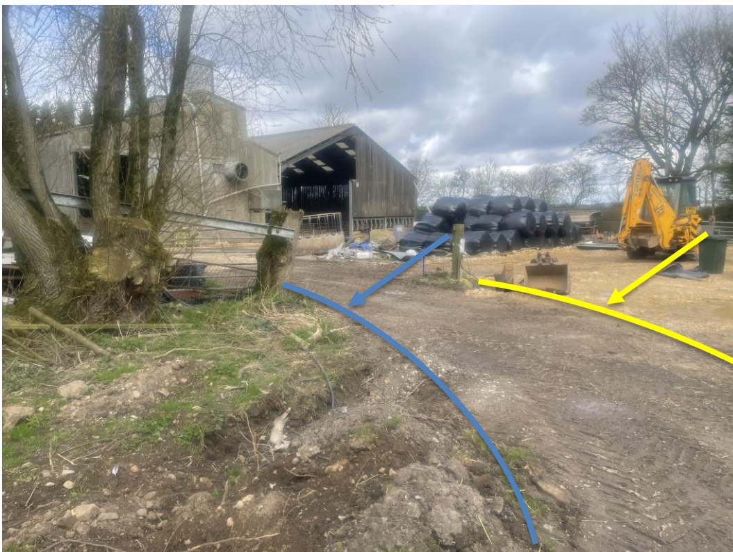
Image 10 – Heavily compacted access track (blue) and south extent of previous excavations is indicated (yellow).
