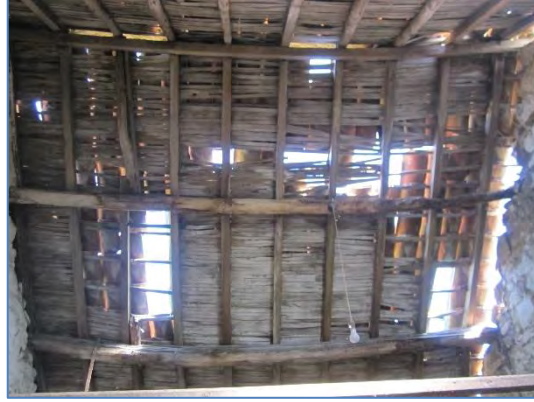
Photo 12: Building B-Eastern section.
