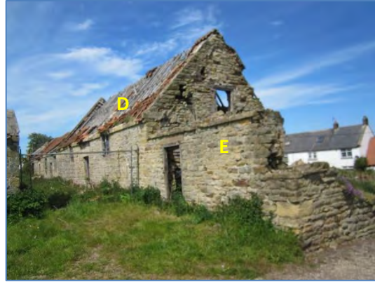
Photo 2: Buildings A to E taken from east.
