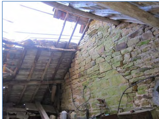
Photo 10: Building B-Western section
