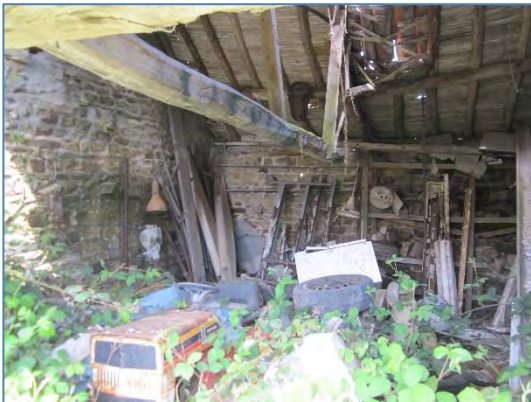
Photo 9: Building B-western section.
