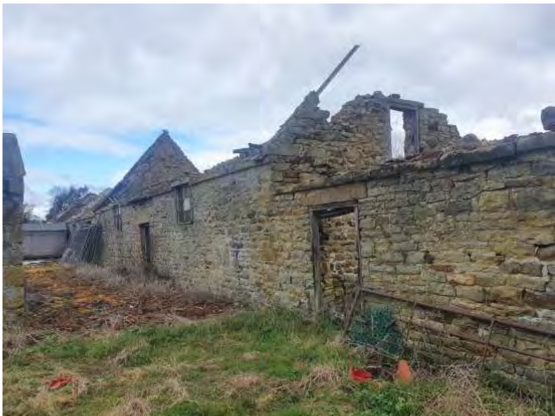
Photo 3. Rear view of the traditional buildings.
