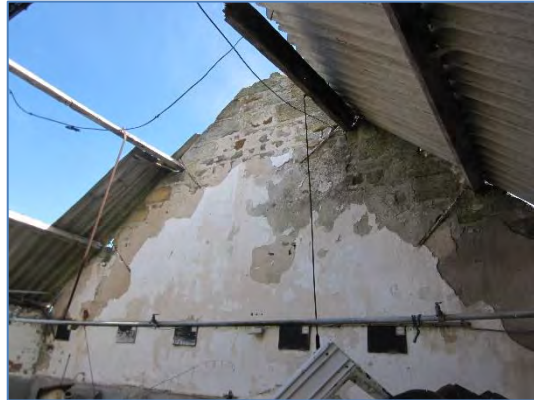
Photo 6: Building A – Internal roof.
