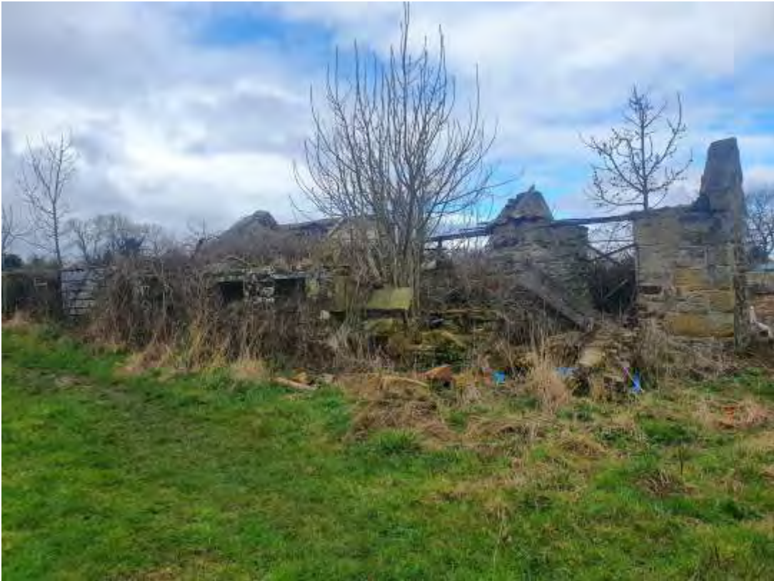
Photo 6. Pigsty's and store to rear of the main block of buildings.
