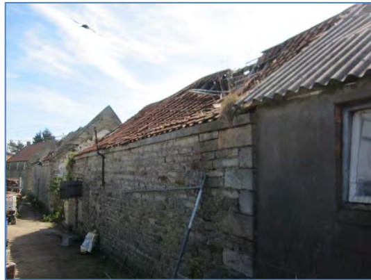
Photo 8: Building B – north side.
