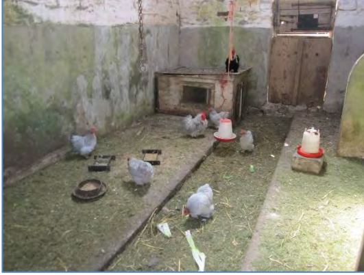
Photo 11: Building B – Eastern section.
