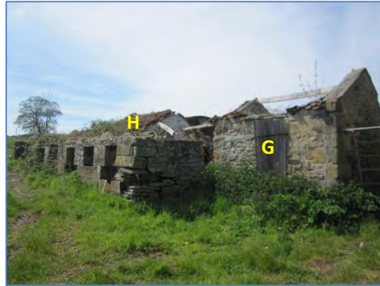
Photo 4: Building G and H
