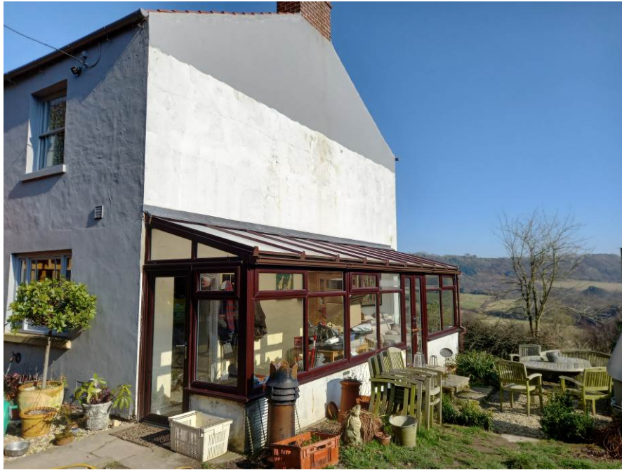
This photograph shows the side elevation of Darncombe Farm and the existing fully glazed lean-to garden room extension.
