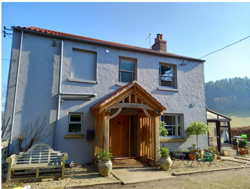
This photograph shows the front elevation of Darncombe Farm and the timber and pantile porch, which is included in this scheme for retrospective planning consent.
