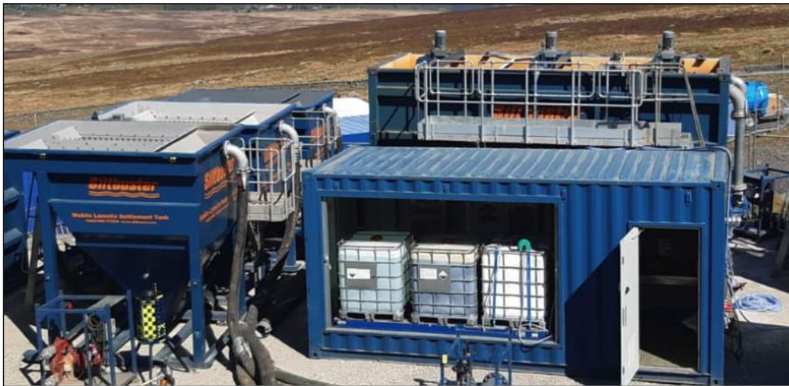
Image 14 – 120m 3 /hr Siltbuster, a similar unit will be used at Ladycross.
