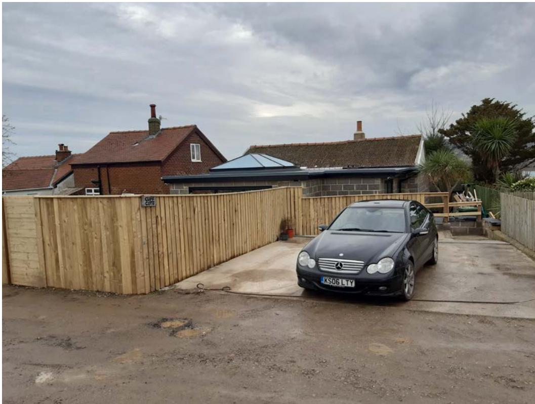
View of Cliff Cote from Prospect Field showing the neighbouring properties to either side
