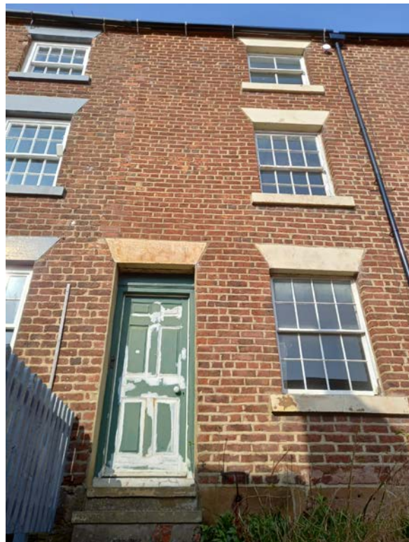
This photograph shows the front elevation of 3 The Esplanade.
