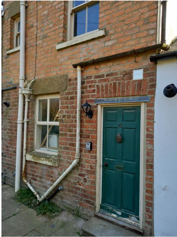
This photograph shows the rear elevation of 3 The Esplanade.
