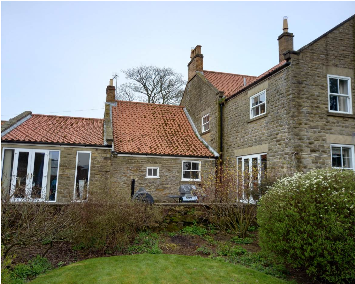
This photograph shows the rear elevation of Broxa Farmhouse and the proposed siting of the garden room.
