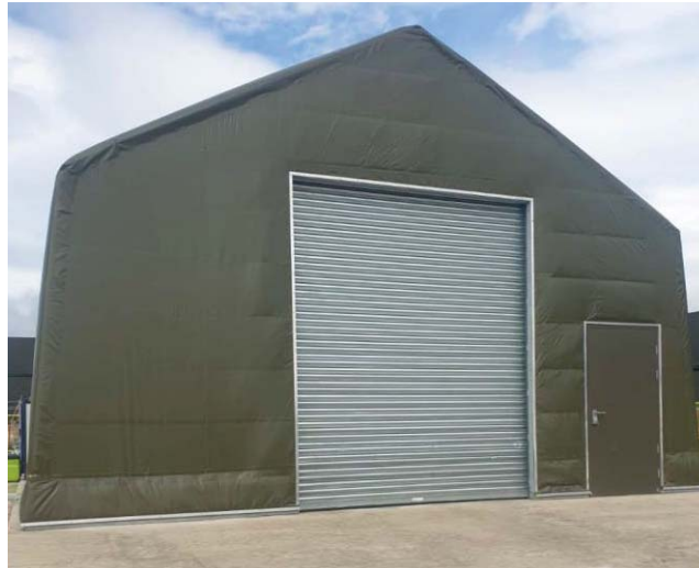
Figure 2: Additional storage and covered bay structure
