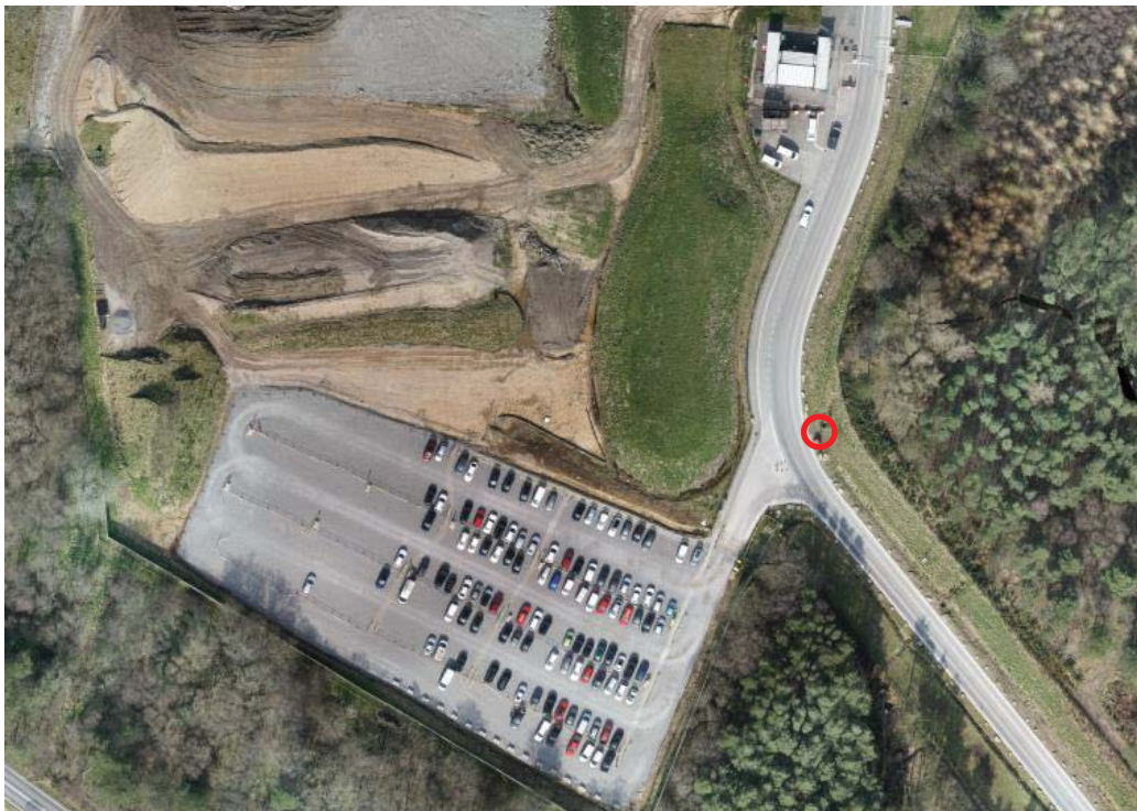
Figure 1: Location of entrance temporary column light circled in red
