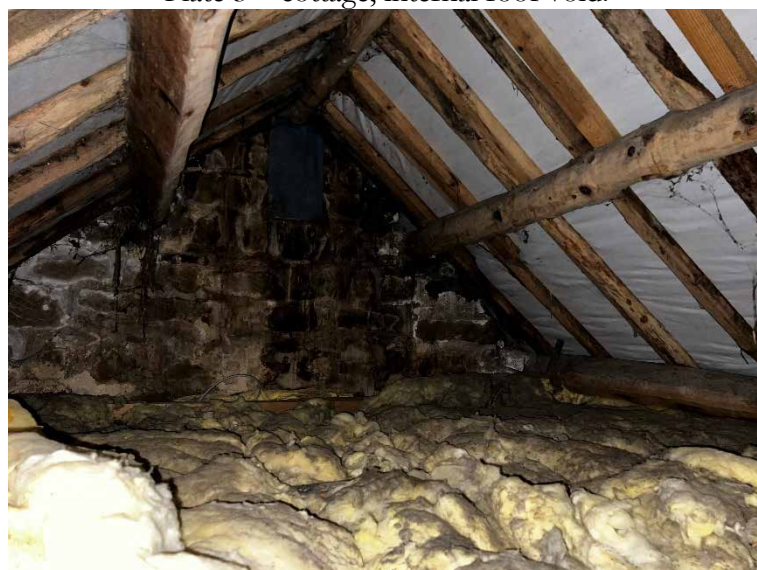
Plate 3 – cottage, internal roof void.
