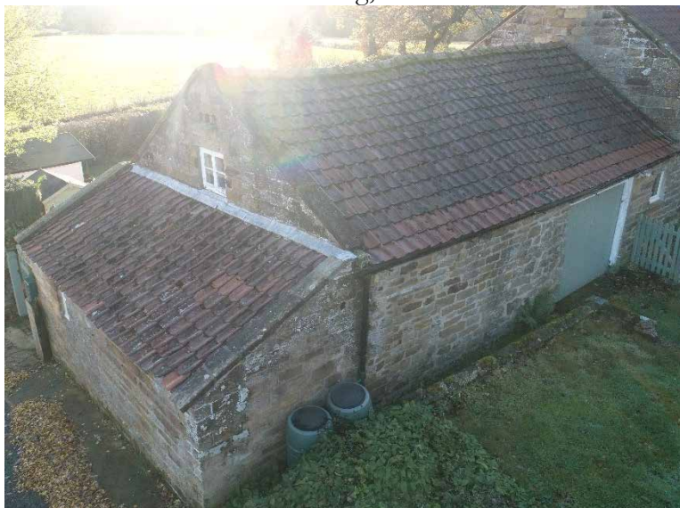
Plate 5 – outbuilding, south elevation and east gable.
