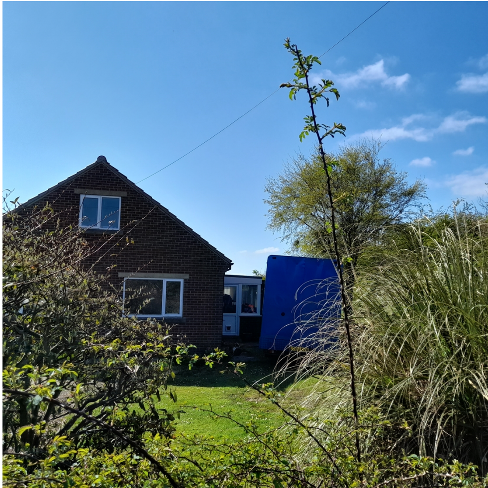
View from public highway to north
