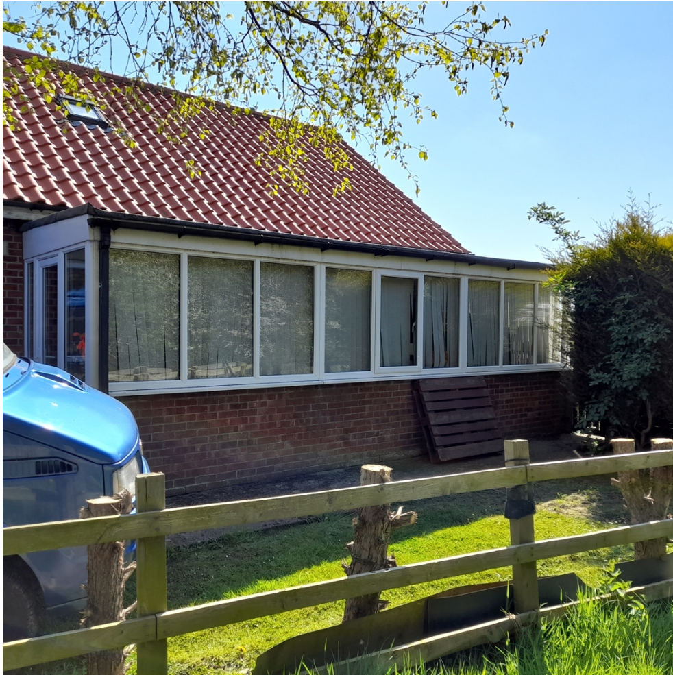
View from field access track to west
