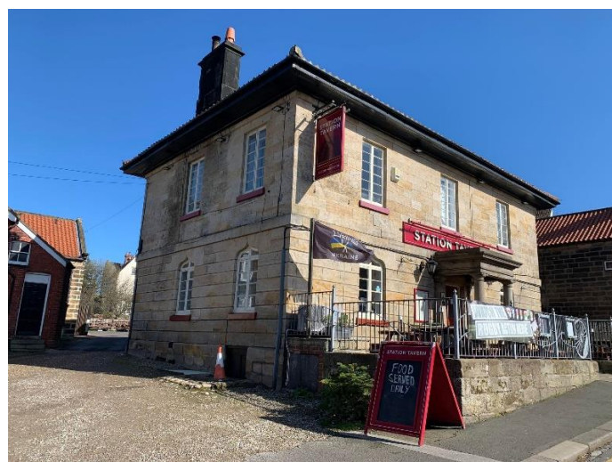
Photos above showing the location of the existing cooling unit to the front left side of the building.
