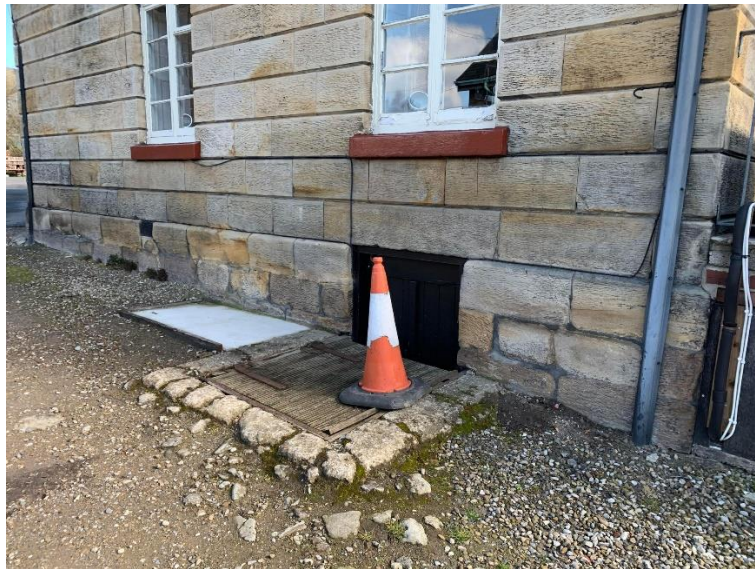
Photo showing the west side elevation and existing ground floor windows.
