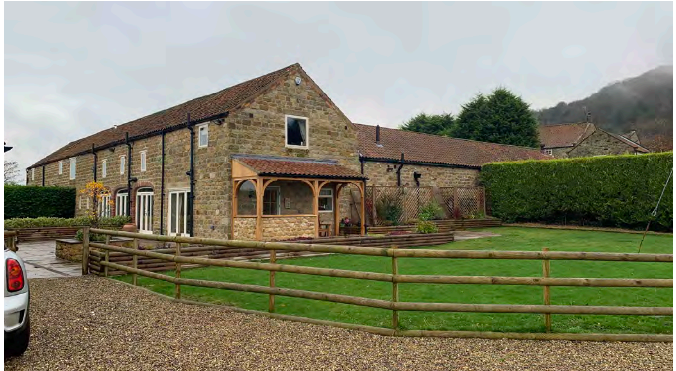
Arrival and north east side of barn
