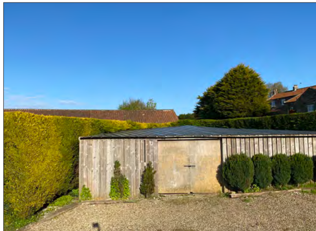
View of shed
