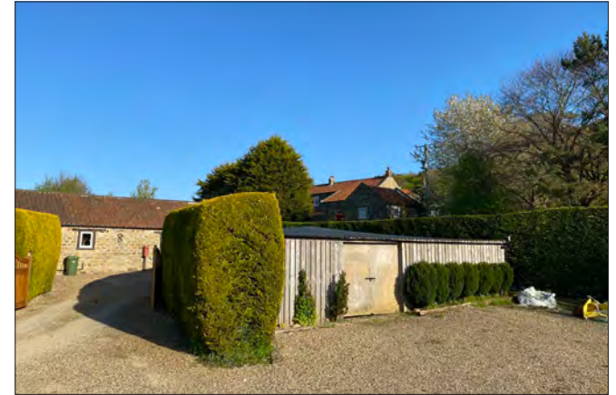
Timber shed from west
