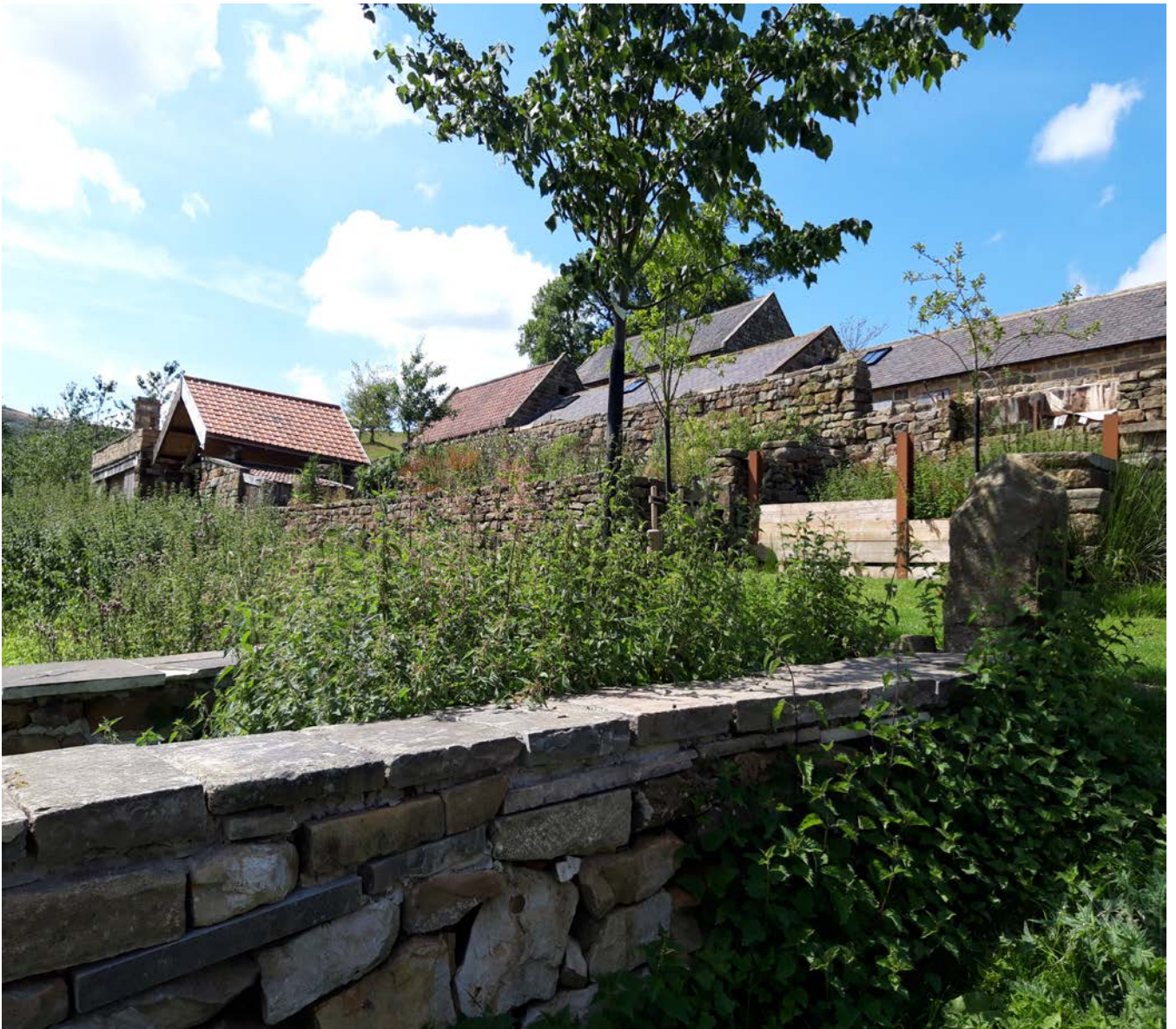
Wider shot of 'High Barns' Buildings.
