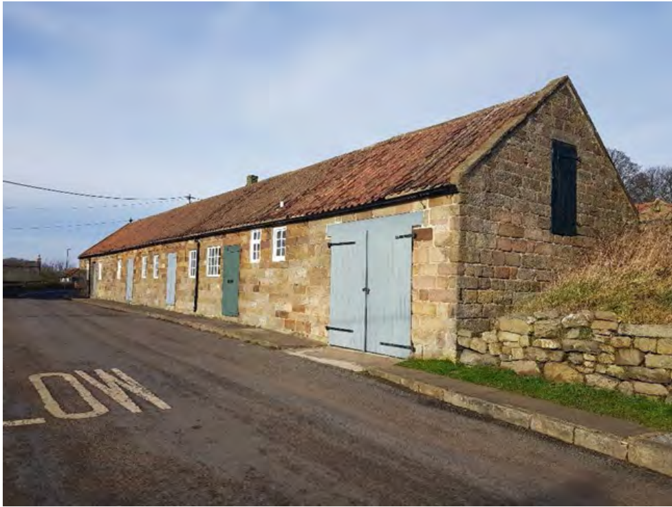
Photo 9 – View of Cross Farm Outbuilding (site is to rear)
