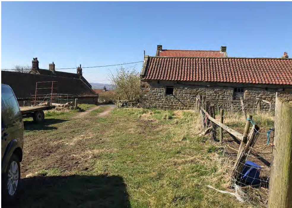
Photo 7 – View of access from site looking west
