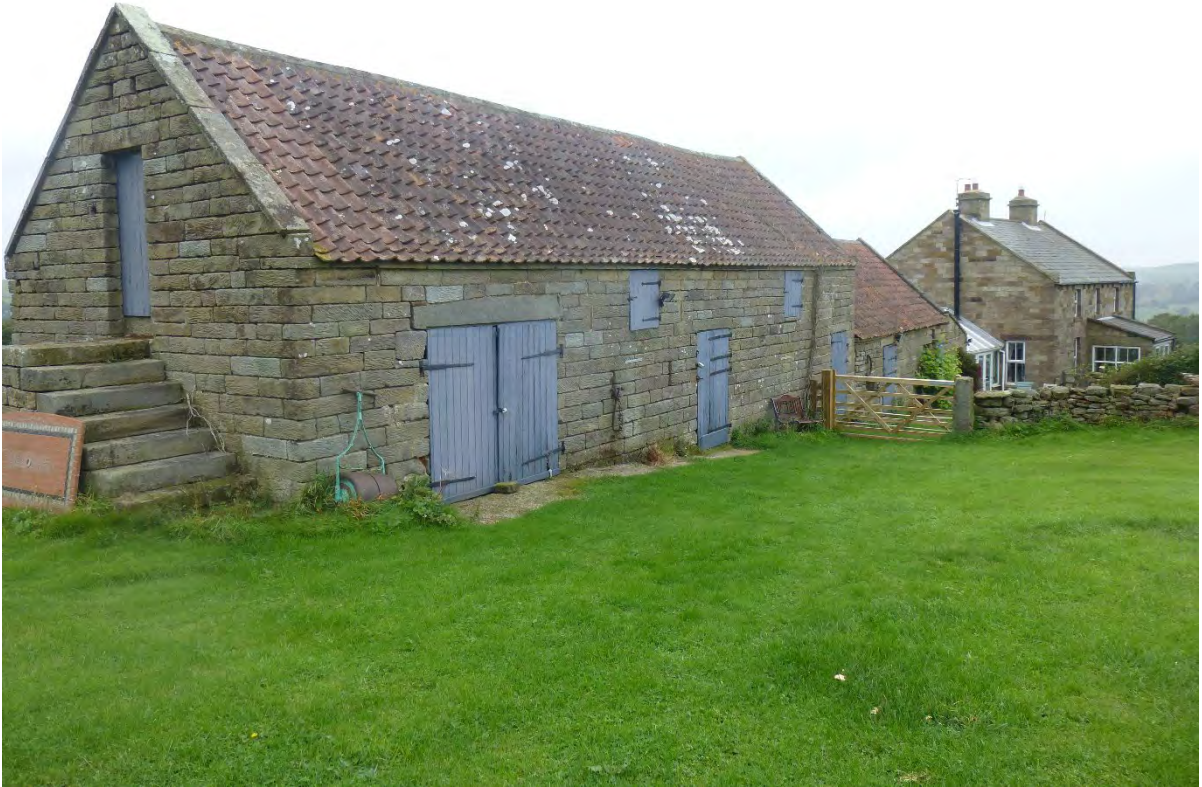
3. View of outbuilding looking northwest from southern garden area
