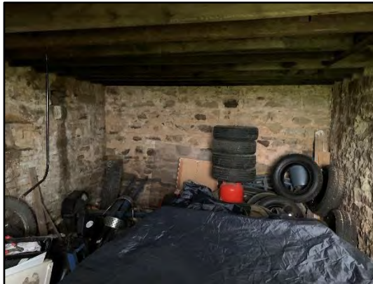
Photo 7: Inside ground floor section of 1a.
