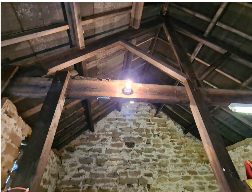
Figure 7: Internal view of Snowdon Nab outbuilding (central section)
