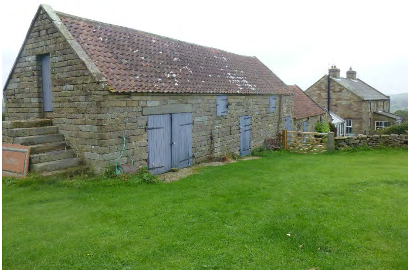
Figure 4: View of outbuilding and adjacent former farmhouse from garden (looking north-west)
