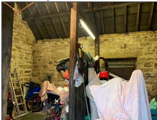
Photo 9: Inside section 1b.
