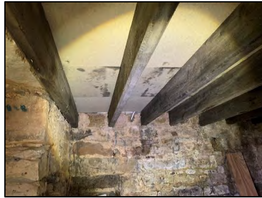
Photo 8: Ceiling of ground floor, section 1a.
