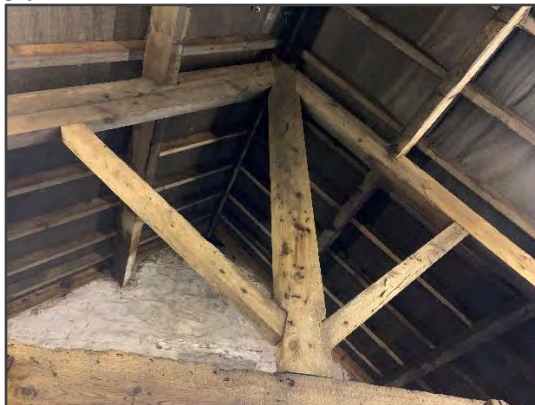
Photo 15: Roof trusses and purlins of section 2a.
