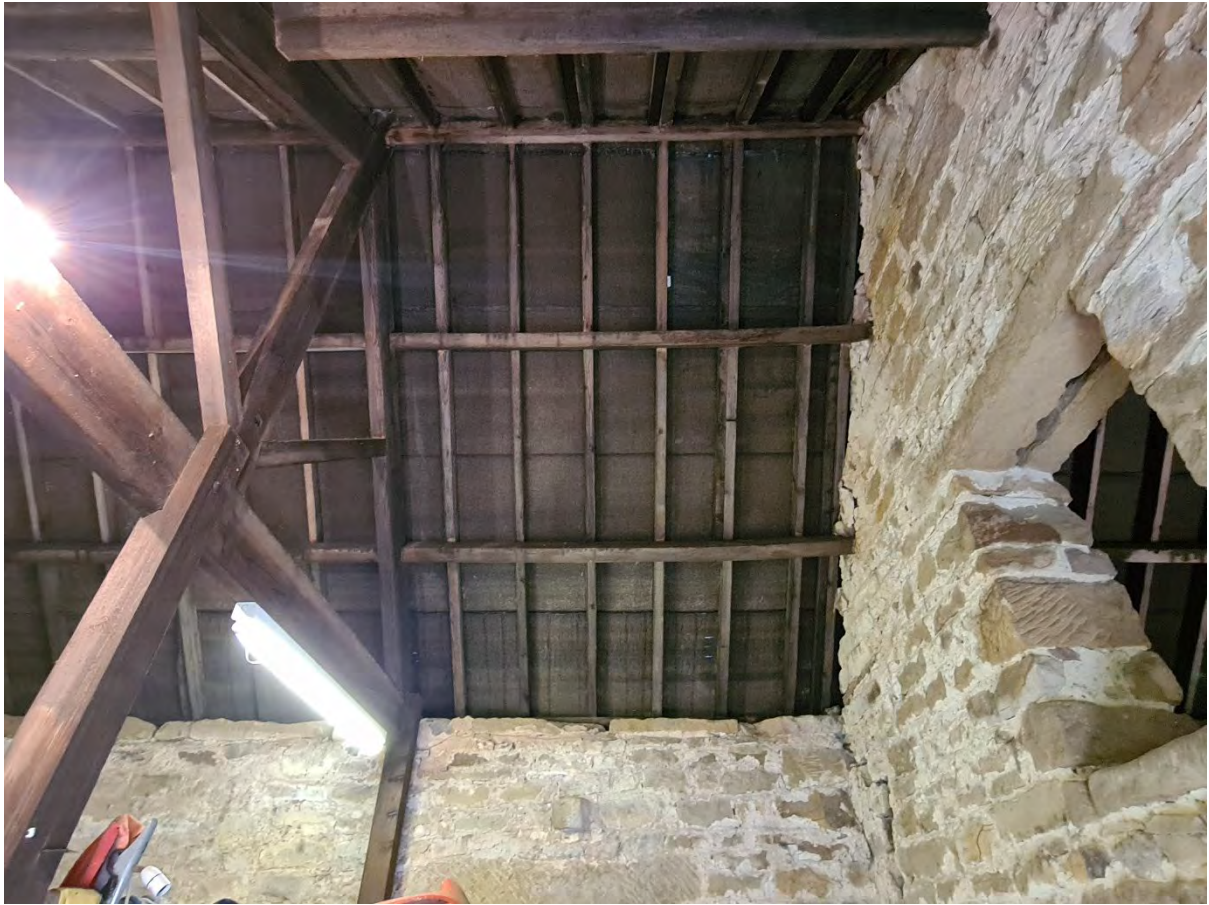
9. View of interior roof rafters
