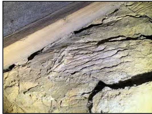
Photo 6: Wall top gaps.
