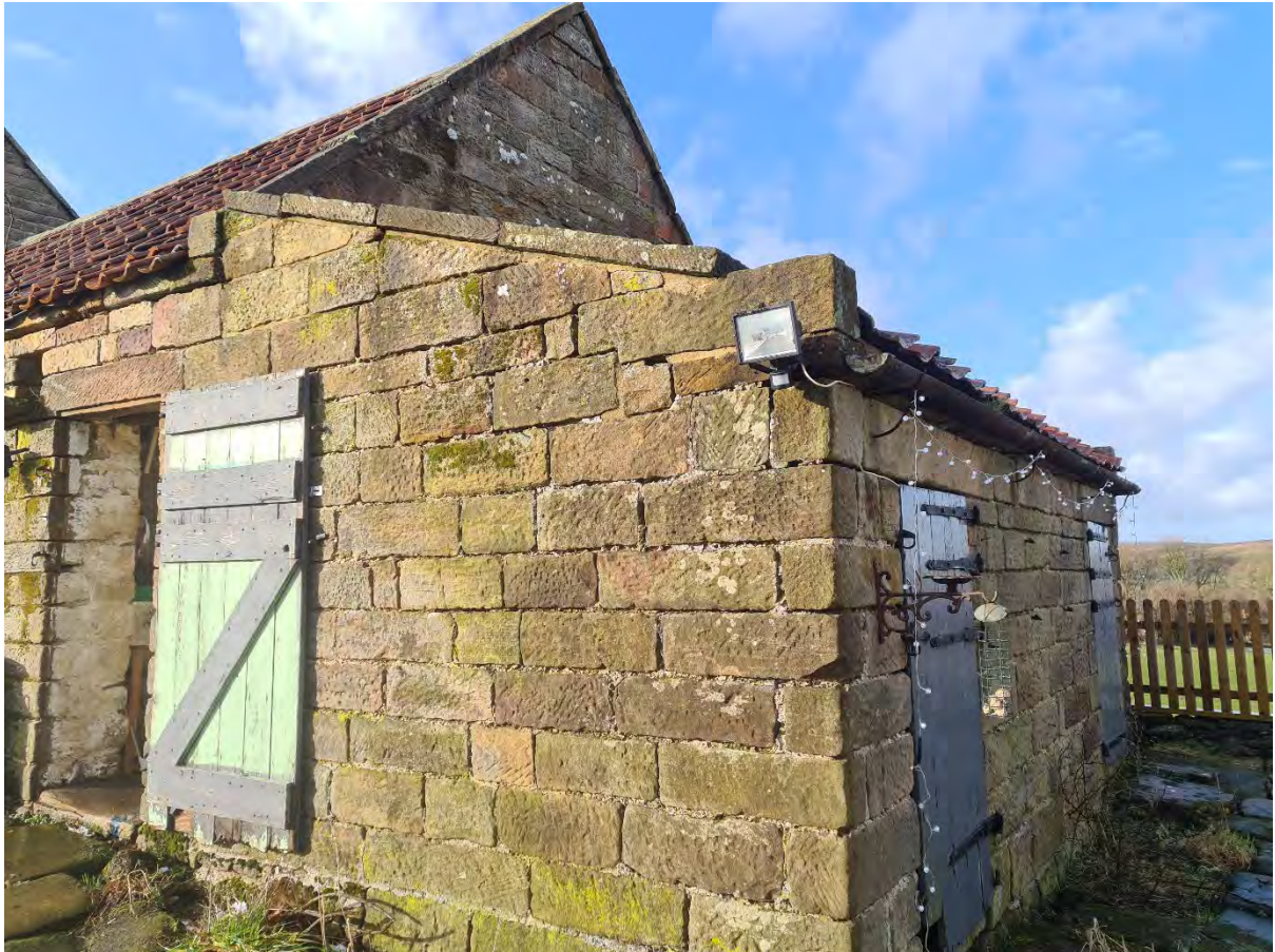
7. View of lean to (northern end of outbuilding)
