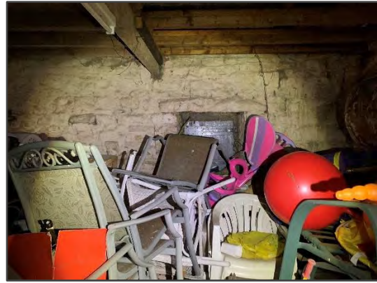
Photo 12: Inside section 1c.
