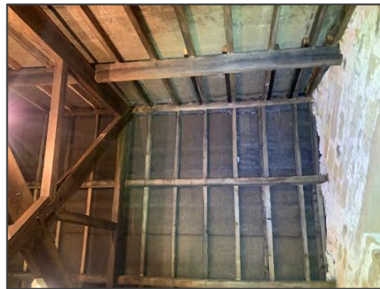
Photo 10: Exposed internal roof ridge with lining.
