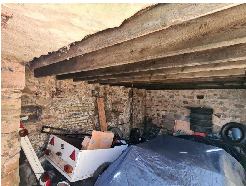
Figure 9: Internal view of Snowdon Nab outbuilding (garage)
