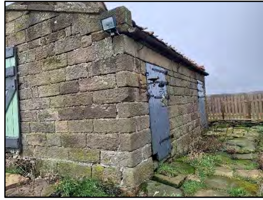
Photo 20: External view of 2c.
