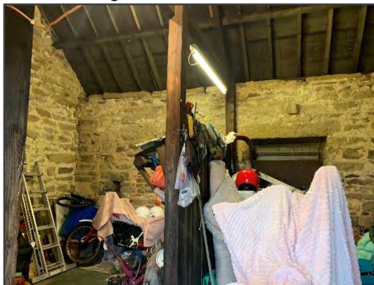
Photo 9: Inside section 1b.
