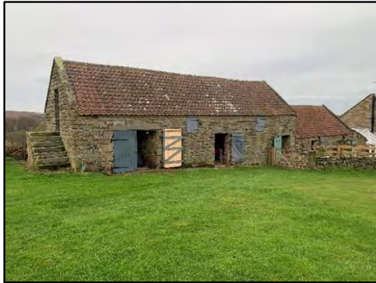
Photo 1: Eastern aspect of the buildings.
