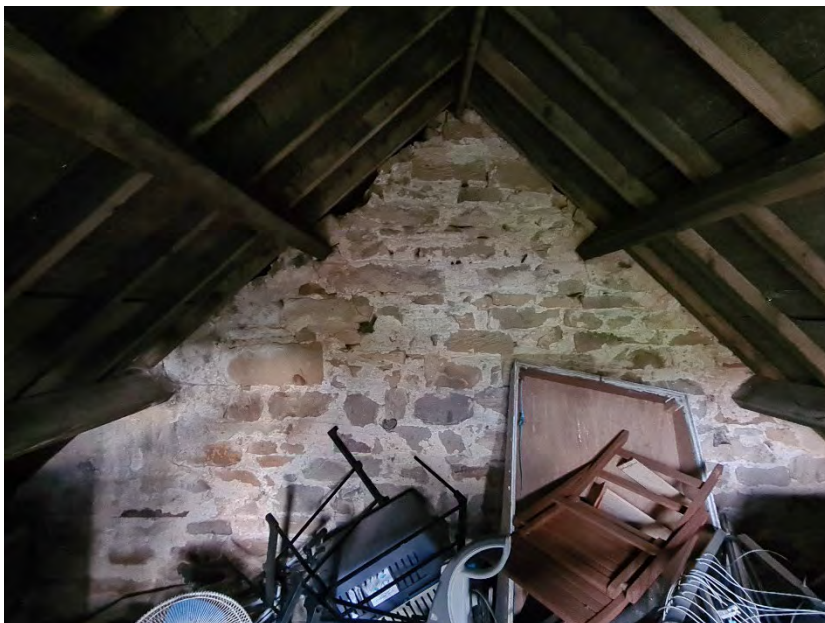
Figure 8: Internal view of Snowdon Nab outbuilding (above garage space)
