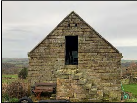
Photo 3: South aspect of the building.
