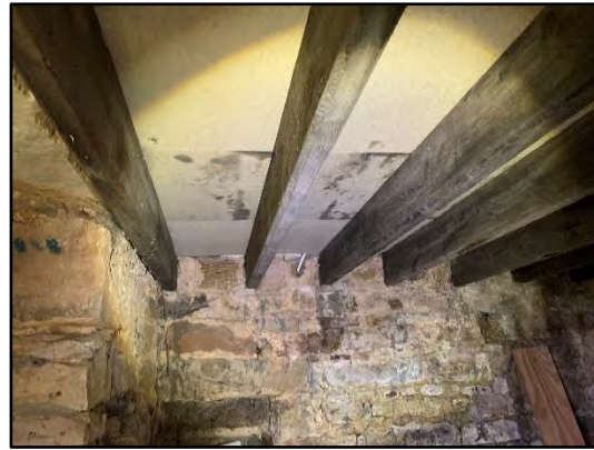
Photo 8: Ceiling of ground floor, section 1a.
