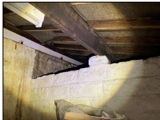
Photo 18: Inside lean-to section of 2c.
