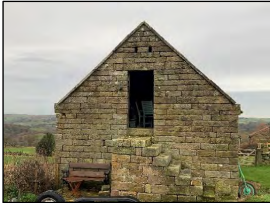
Photo 3: South aspect of the building.
