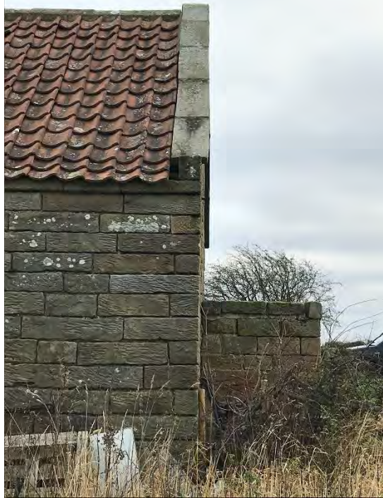
Rear corner of building 1- perpendicular Gable
