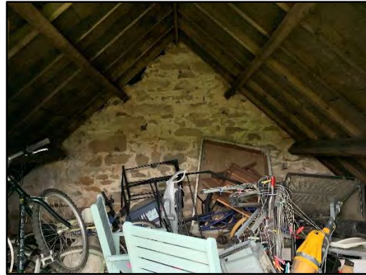
Photo 4: Inside hayloft of section 1a.
