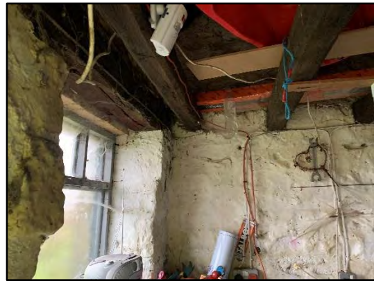
Photo 16: Internal view of section 2b.
