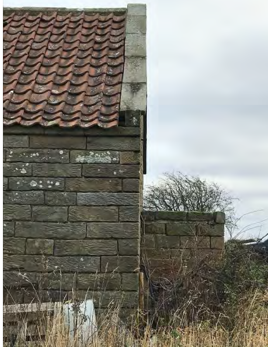
Rear corner of building 1- perpendicular Gable
