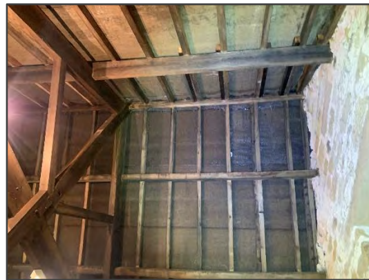
Photo 10: Exposed internal roof ridge with lining.
