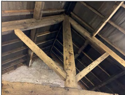
Photo 15: Roof trusses and purlins of section 2a.
