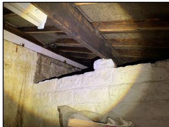
Photo 18: Inside lean-to section of 2c.
