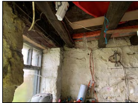
Photo 16: Internal view of section 2b.
