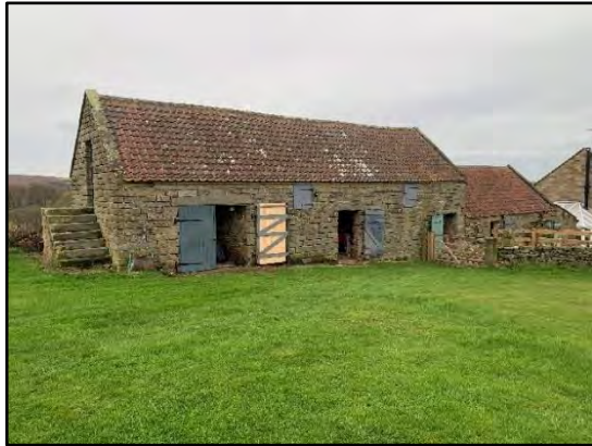
Photo 1: Eastern aspect of the buildings.
