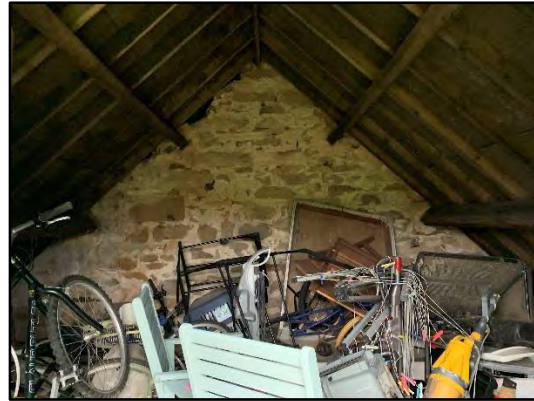
Photo 4: Inside hayloft of section 1a.
