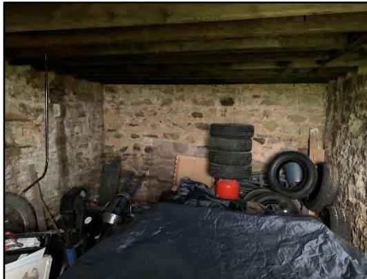
Photo 7: Inside ground floor section of 1a.
