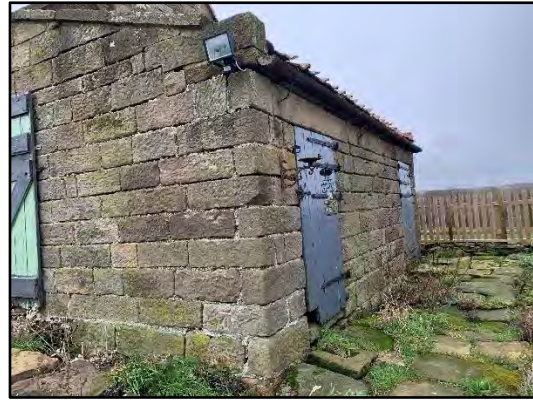
Photo 20: External view of 2c.
