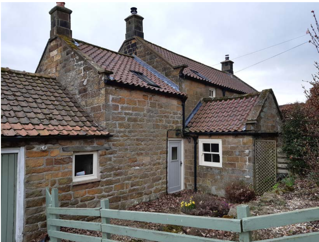
Photo showing the north elevation of South View with the single storey out-shut to be replaced with two storey gabled extension and single storey cat slide extension
