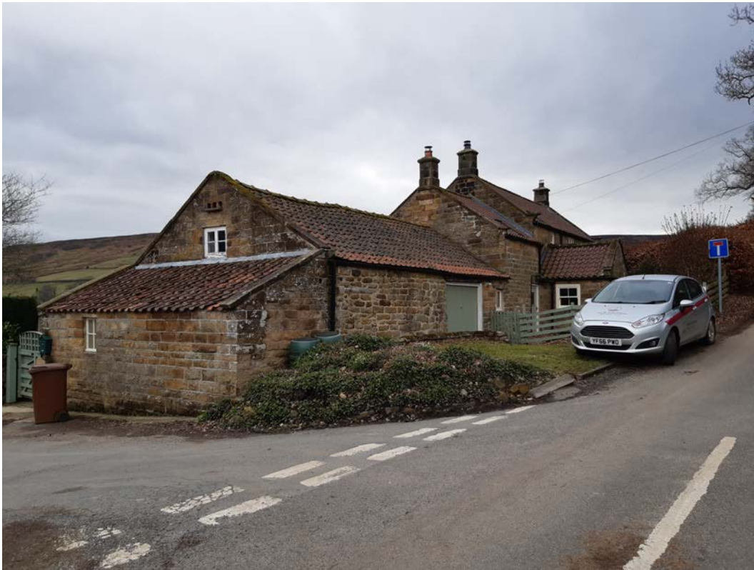
Photo showing the north elevation of South View with the single storey out-shut to be replaced with two storey gabled extension and single storey cat slide extension
