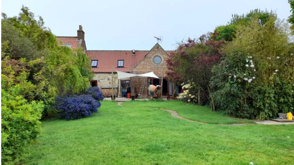
View looking towards the rear elevation and the gabled off shut for which the proposal relates
