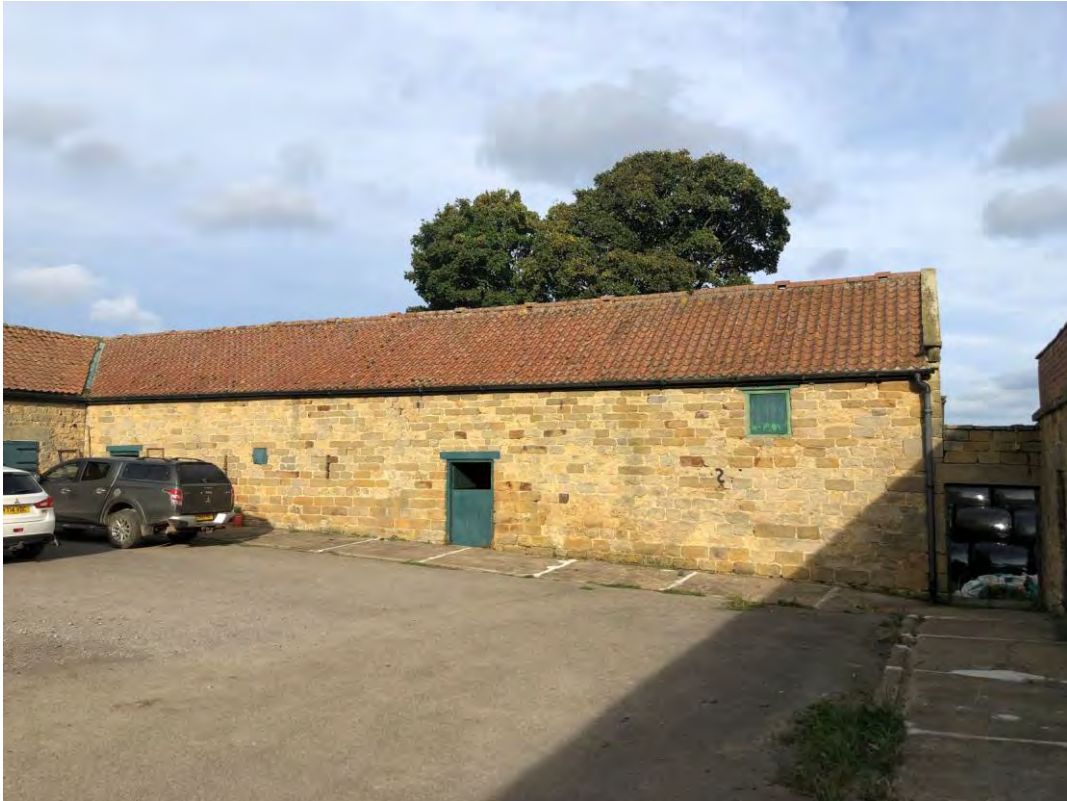
Photograph 1 West elevation, into Farmyard
