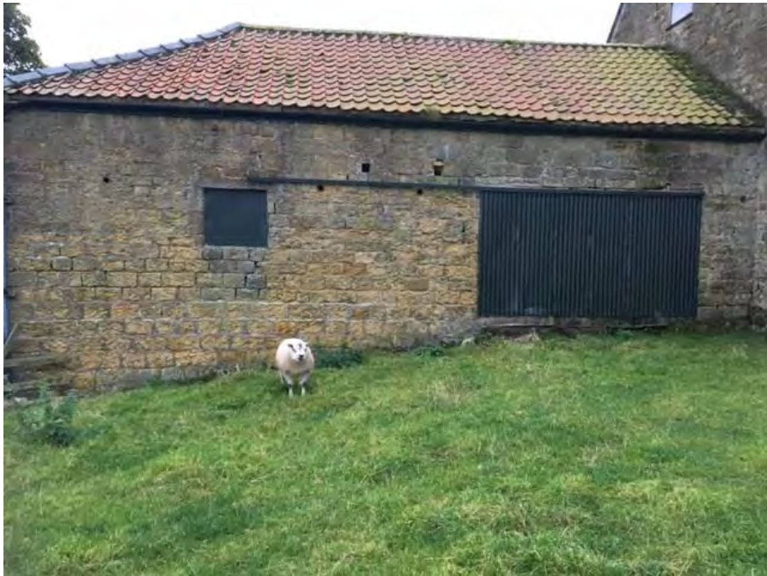
Photograph 5 North elevation abutting farmhouse
