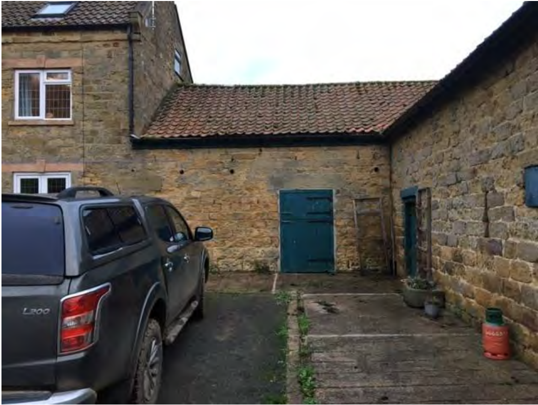
Photograph 2 South elevation abutting farmhouse
