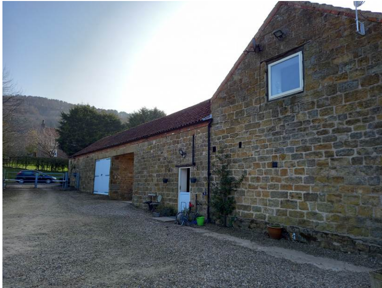
Photograph showing the east elevation of Raincliffe Barn and the carport opening.
