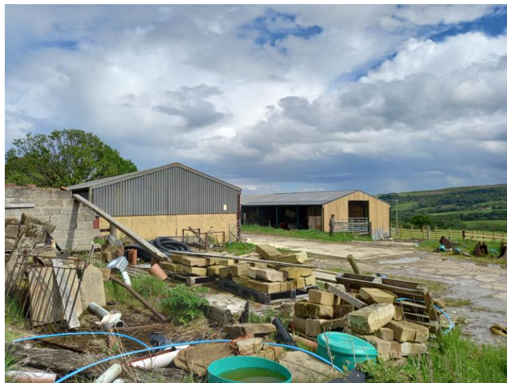
This photograph looks towards the south and shows the existing modern agricultural buildings at Bank House Farm.
