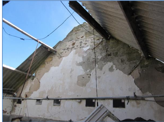
Photo 10: Building A – Internal roof.
