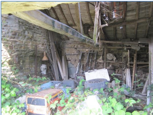
Photo 13: Building B-western section.
