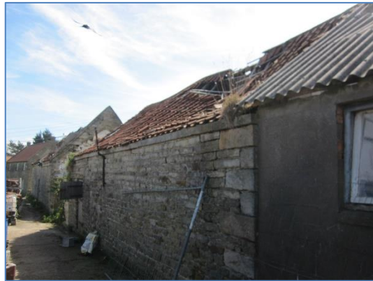
Photo 12: Building B – north side.
