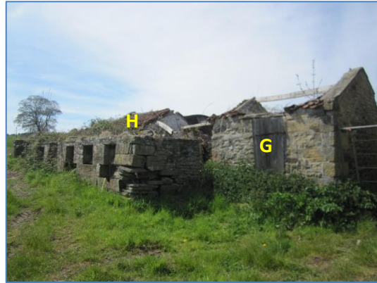
Photo 4: Building G and H
