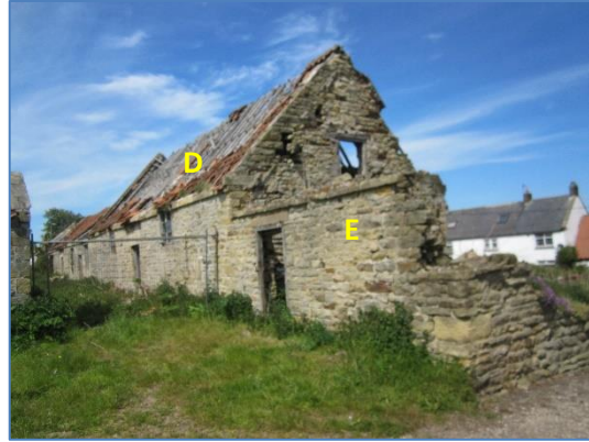
Photo 2: Buildings A to E taken from east.
