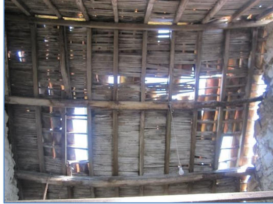
Photo 16: Building B-Eastern section.
