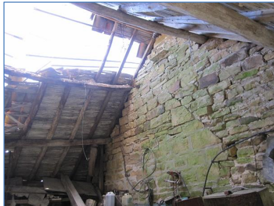
Photo 14: Building B-Western section
