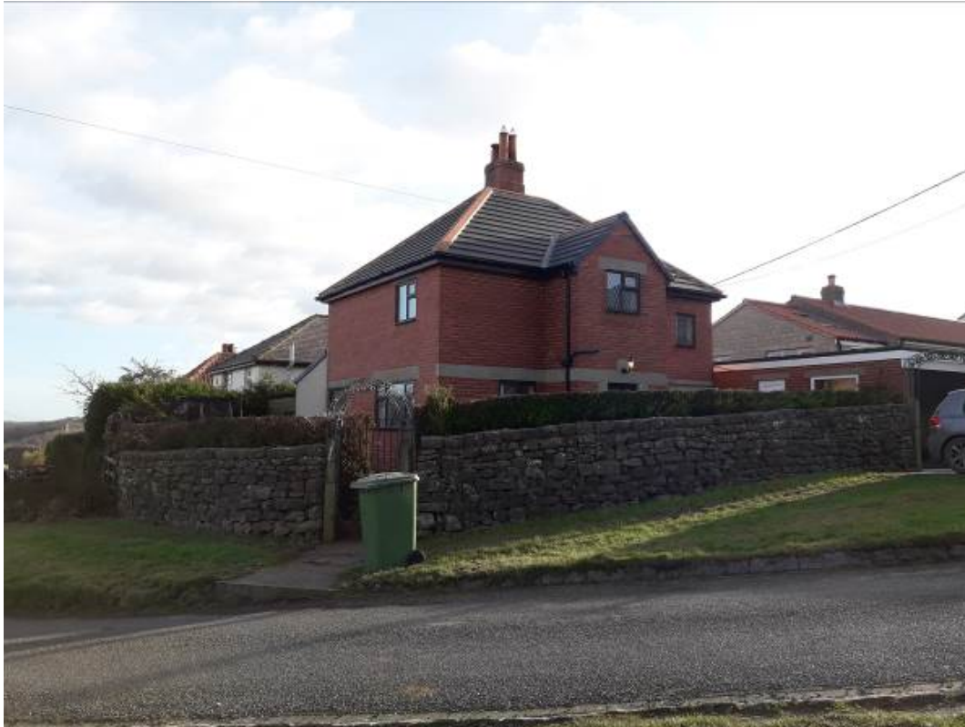
Rear elevation of Heather Lea
