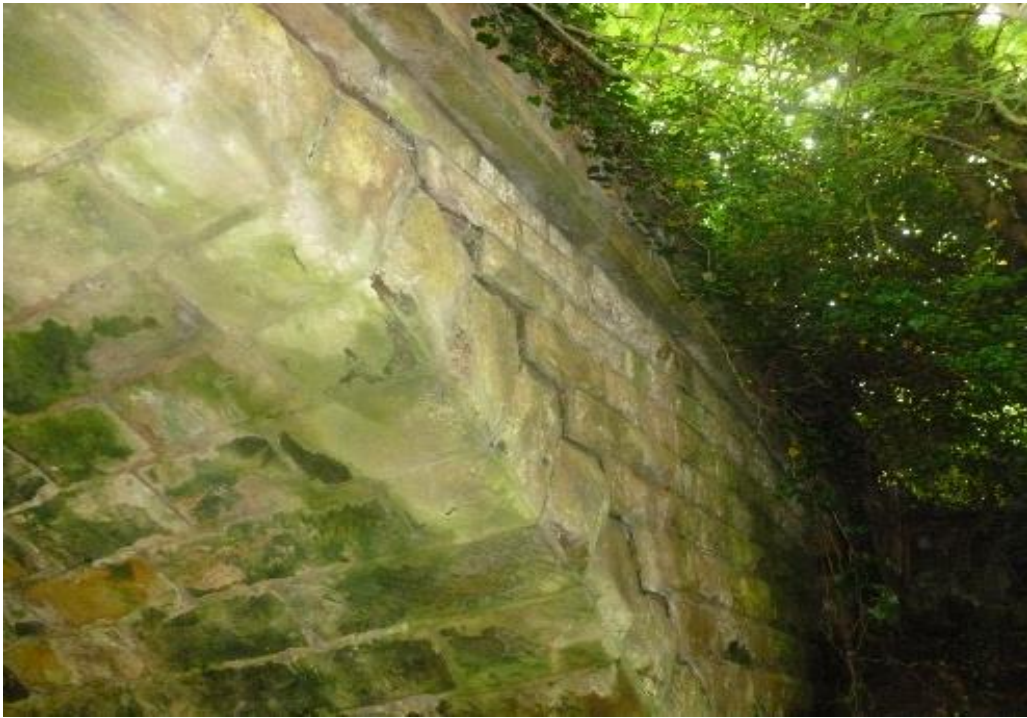
Downstream Elevation (SW Spandrel) - 2015
