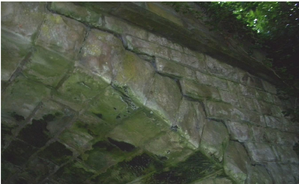
Downstream Elevation (SW Spandrel) - 2011
