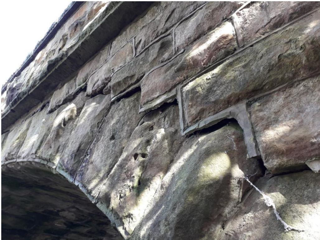
Downstream Elevation (SW Spandrel) – 2021
