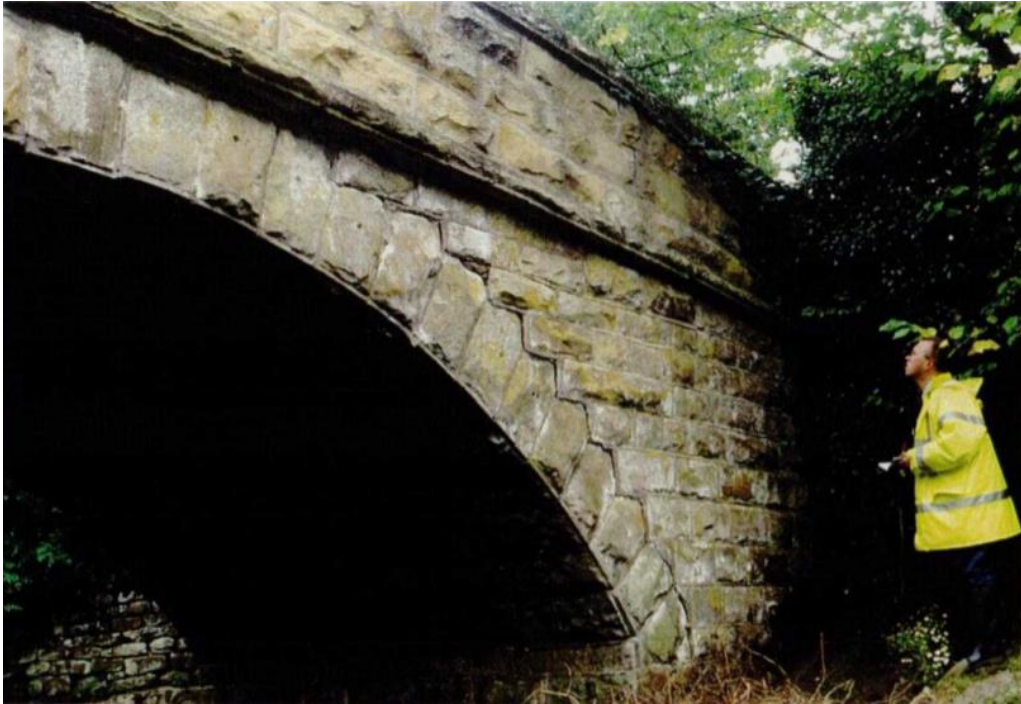
Downstream Elevation (SW Spandrel) – 1997
