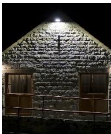
Shielded warm white lights with appropriate controls provide directed light only where and when it is needed.
