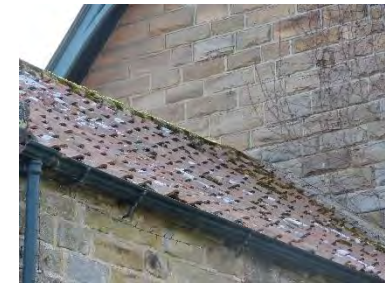
Photo 20. Roof, northern aspect
