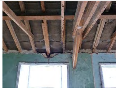
Photo 9: First floor, wall top
