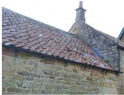
Photo 33. Building roof, northern aspect
