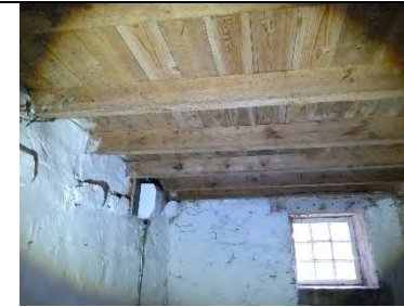
Photo 17: Ground floor, ceiling
