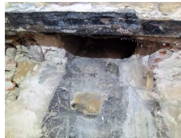
Photo 13: First floor, chimney
