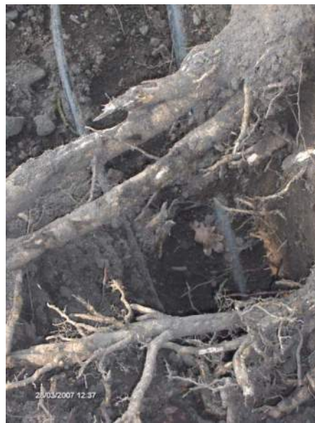
Typical root damage caused by excavation works
