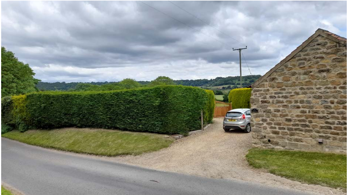
Shed located behind the hedge in foreground – No other views into the site
