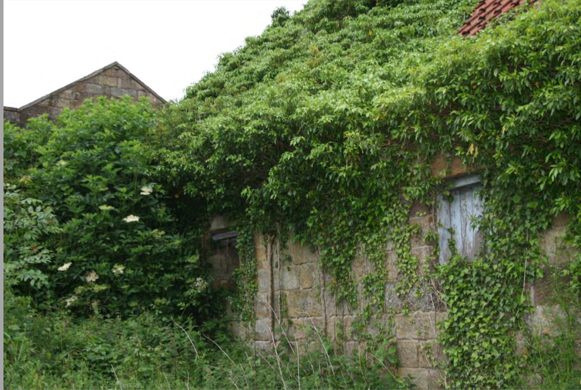
View of Existing Out Barn Looking North East
