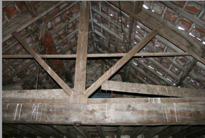
Existing king post trusses
