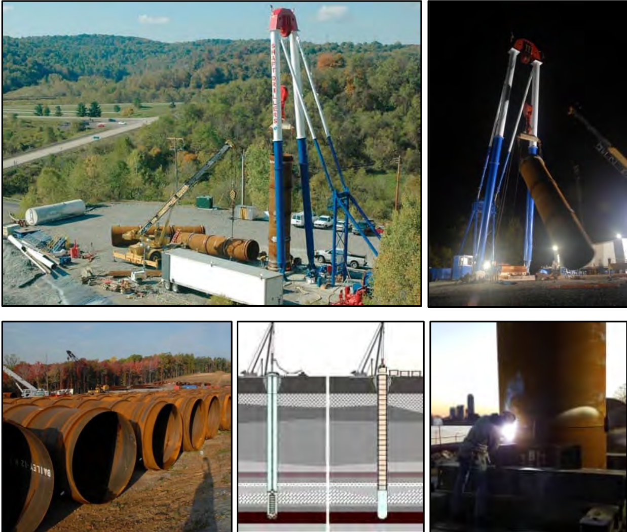
Figure 9: Steel Casing Installation
