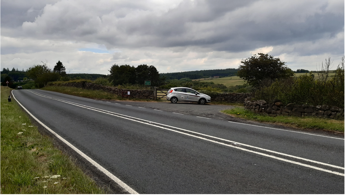
Location of existing access to be closed off with stone wall and grass verge
