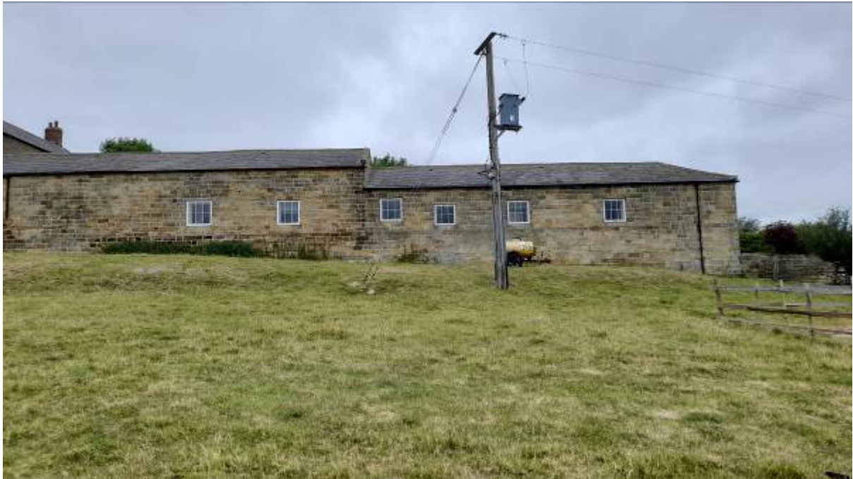
North eastern external elevation
