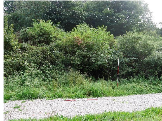
Figure 5: The overgrown earthen bank facing southeast.
