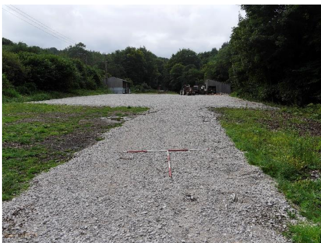
Figure 5: Car park surface (looking west).
