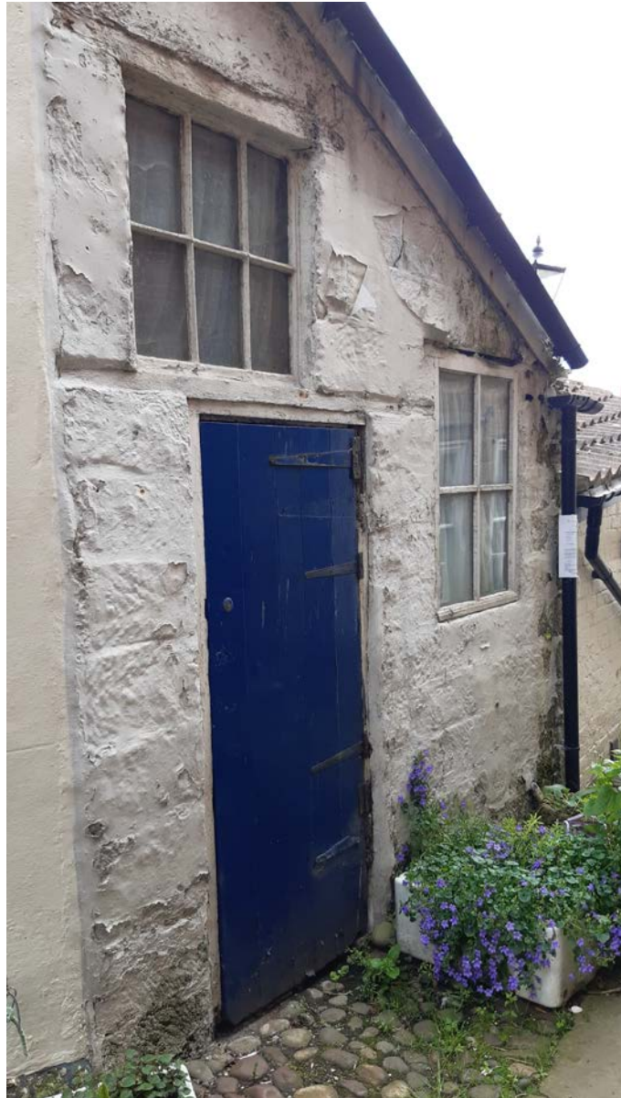
Front elevation of store showing door and windows to be replaced
