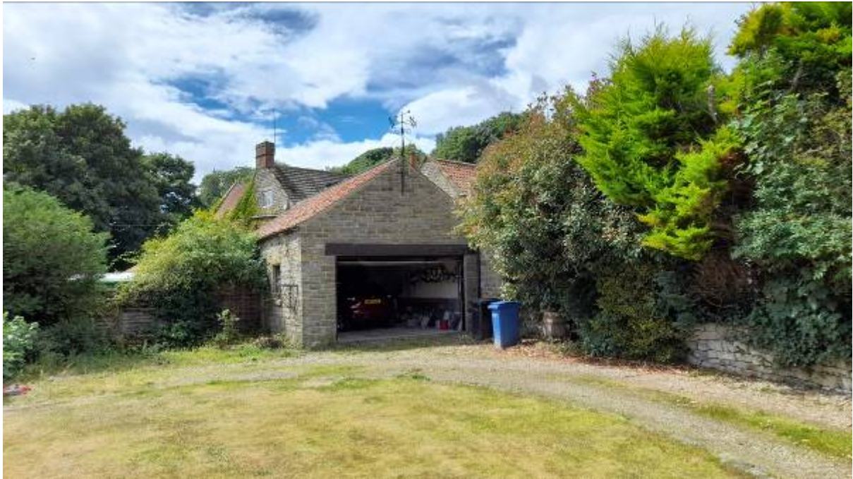
Garage to be converted
