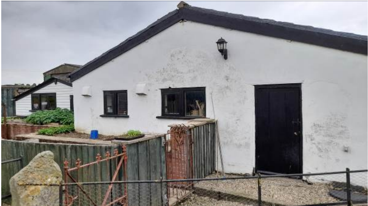
View of southern building of dwelling complex
