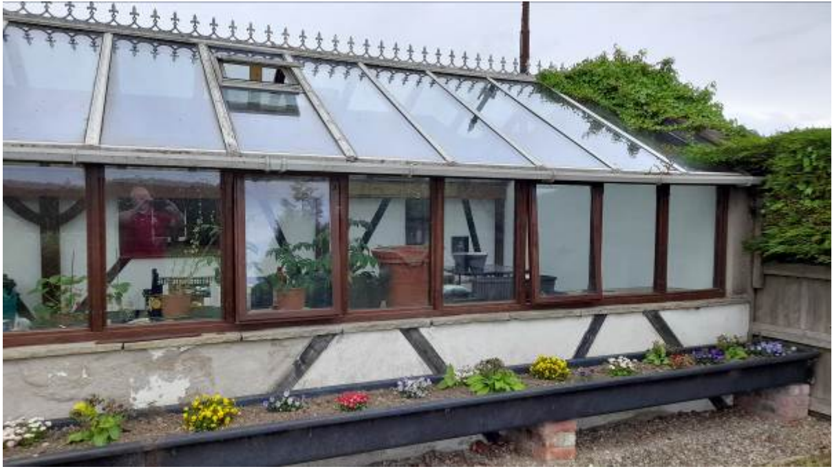
Glass house attached to northern building and boundary with Low Moor Farm
