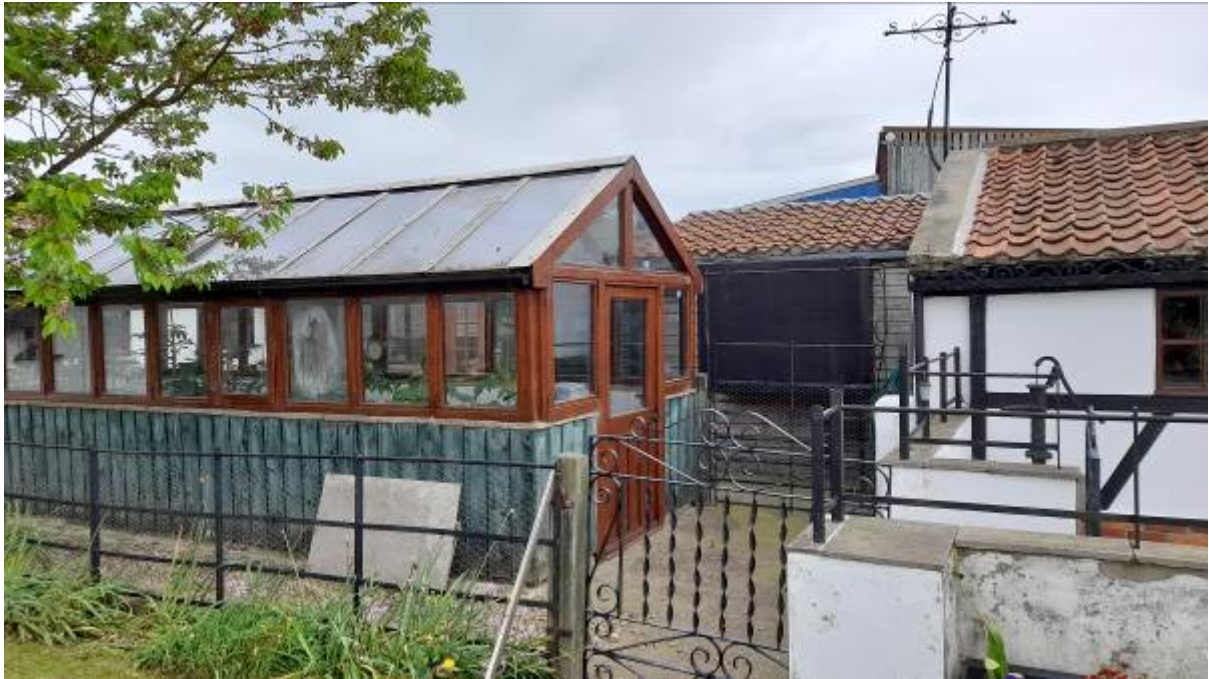
Glass house attached to southern building with northern building in view
