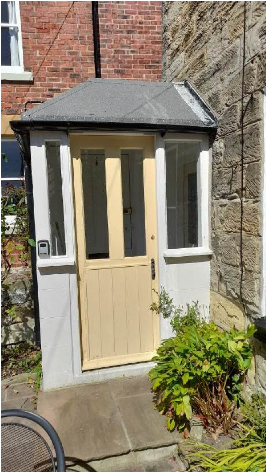
Existing door in rear of modern porch offshut
