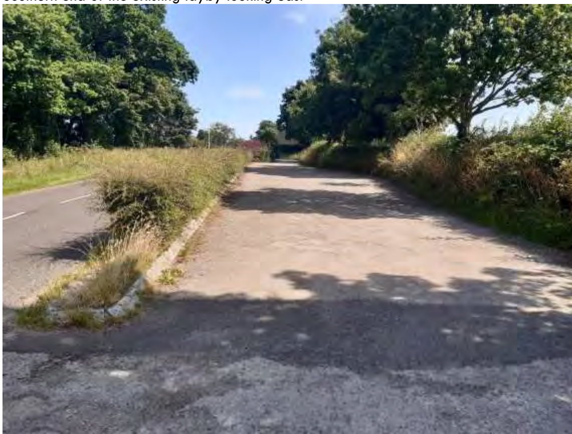
Southern end of layby looking north
