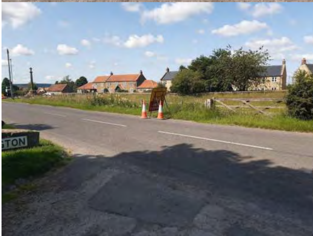
View from southern end of layby looking south
