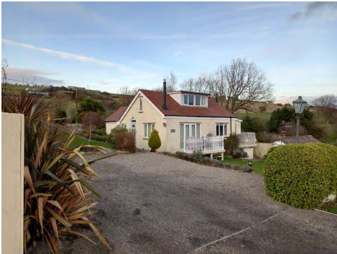
Photo showing front elevation of the property with the dormer and raised decking areas to be replaced
