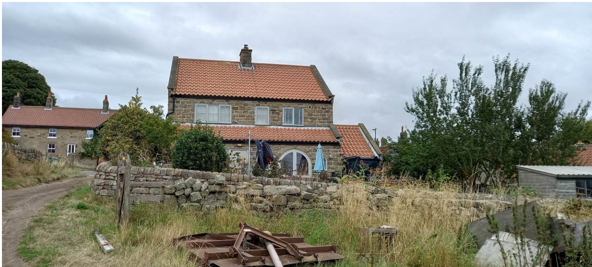
This photograph shows the rear elevation of Milestones, Egton and the siting of the proposed extension.
