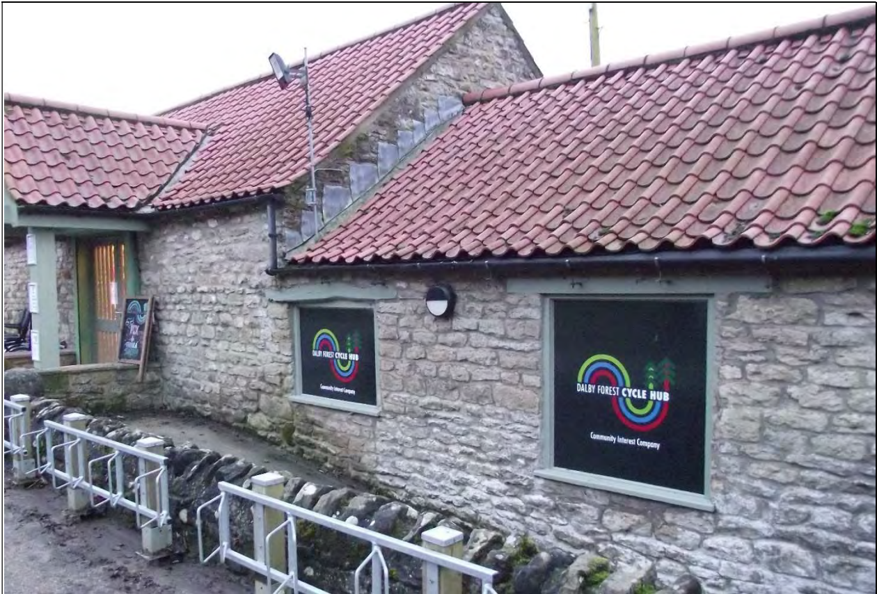
Fittings A & B-Locations at the Cycle Hub from footway/roadway to courtyard
