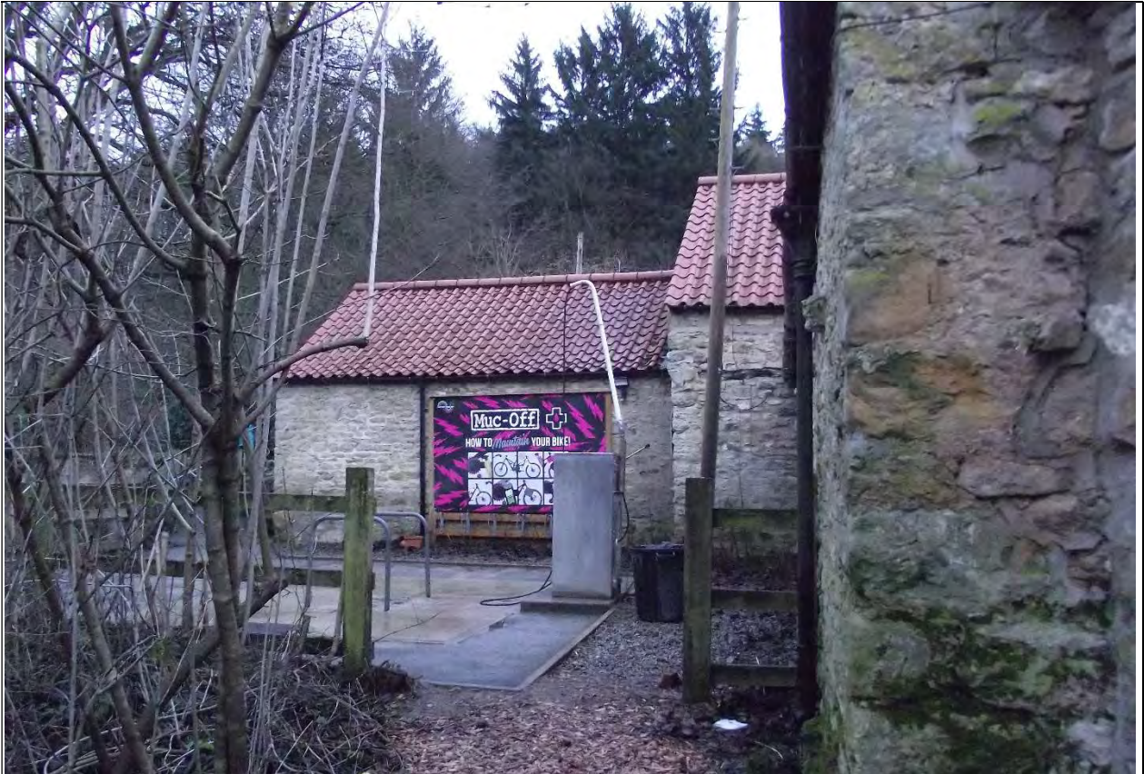
Fitting K-Location at the bike wash area of the Cycle Hub
