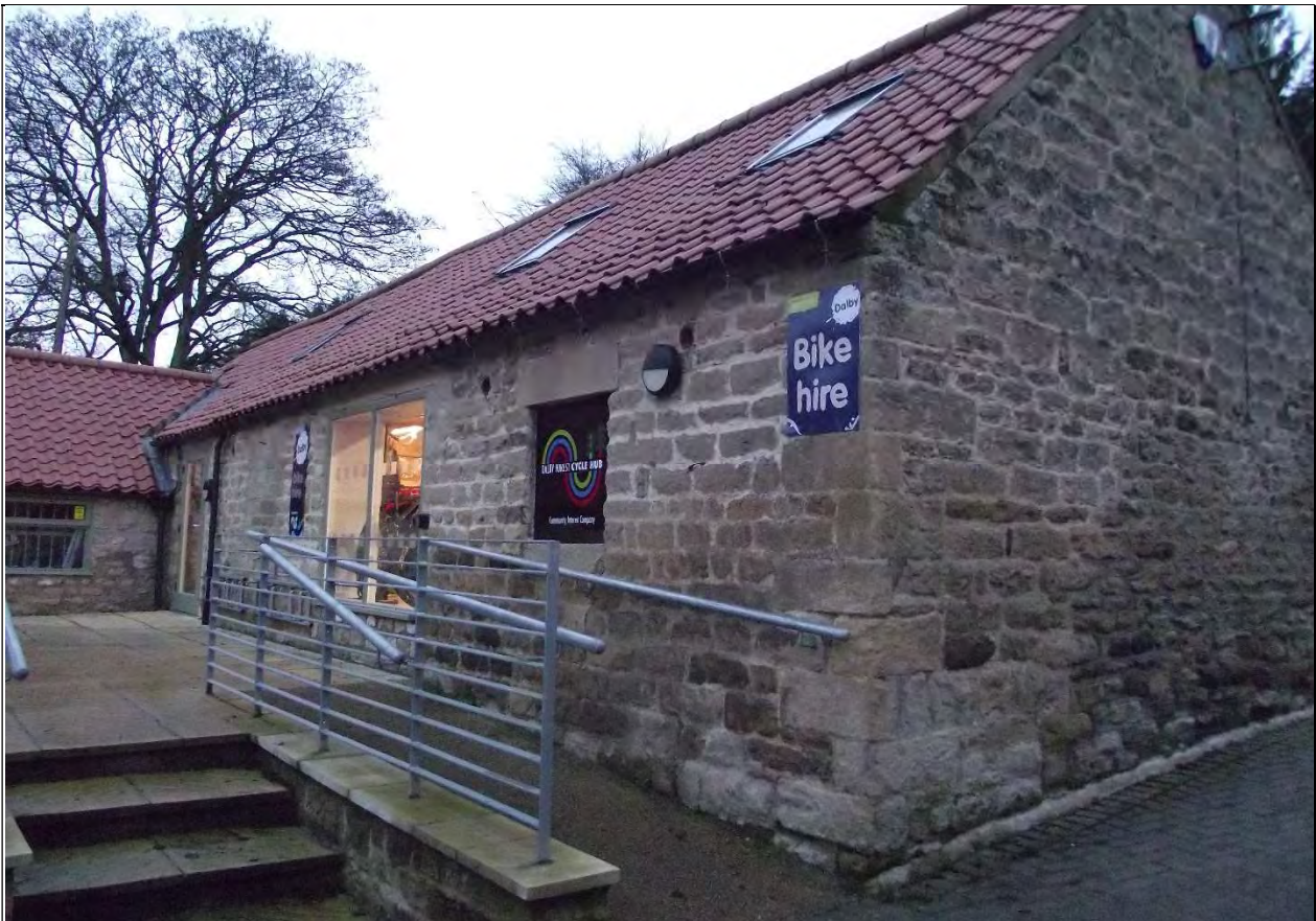
Fittings F & G-Locations at the back of main entrance to the Cycle Hub within the courtyard
