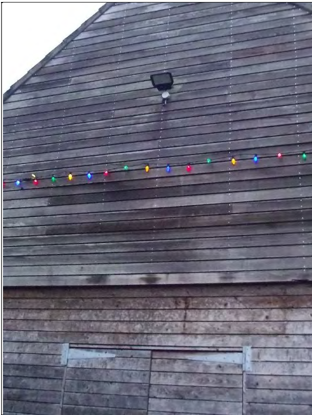
Fittings T-Location on end of building within the courtyard
