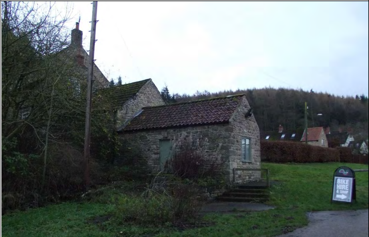
Fitting 1-Location mounted on building opposite cycle hub
