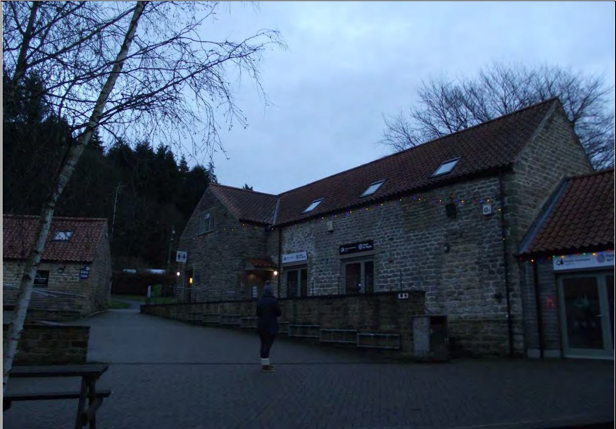
Fittings E, F, M, N & O-Locations on buildings within the courtyard
