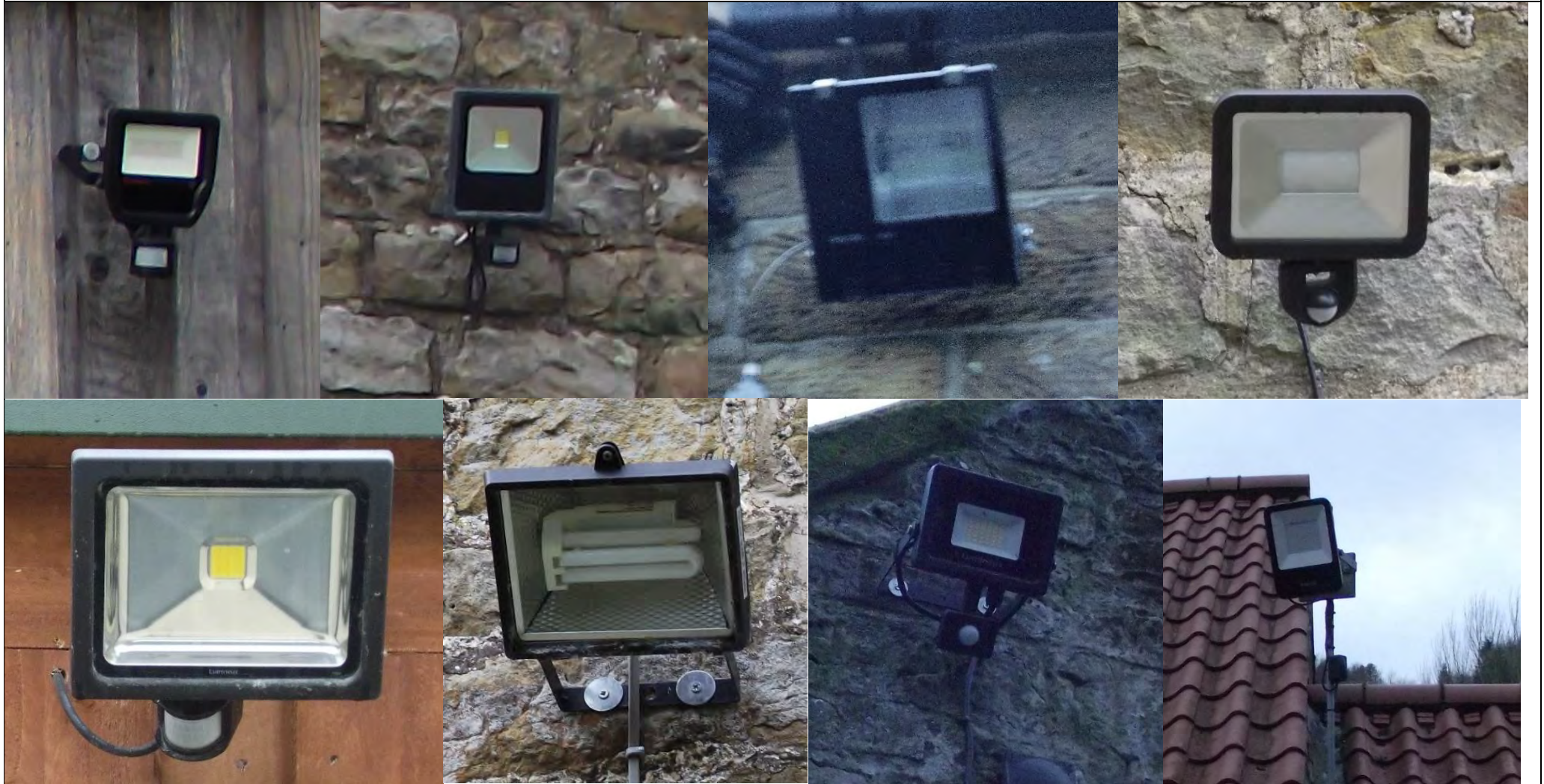
Examples of existing fittings you may find on site
