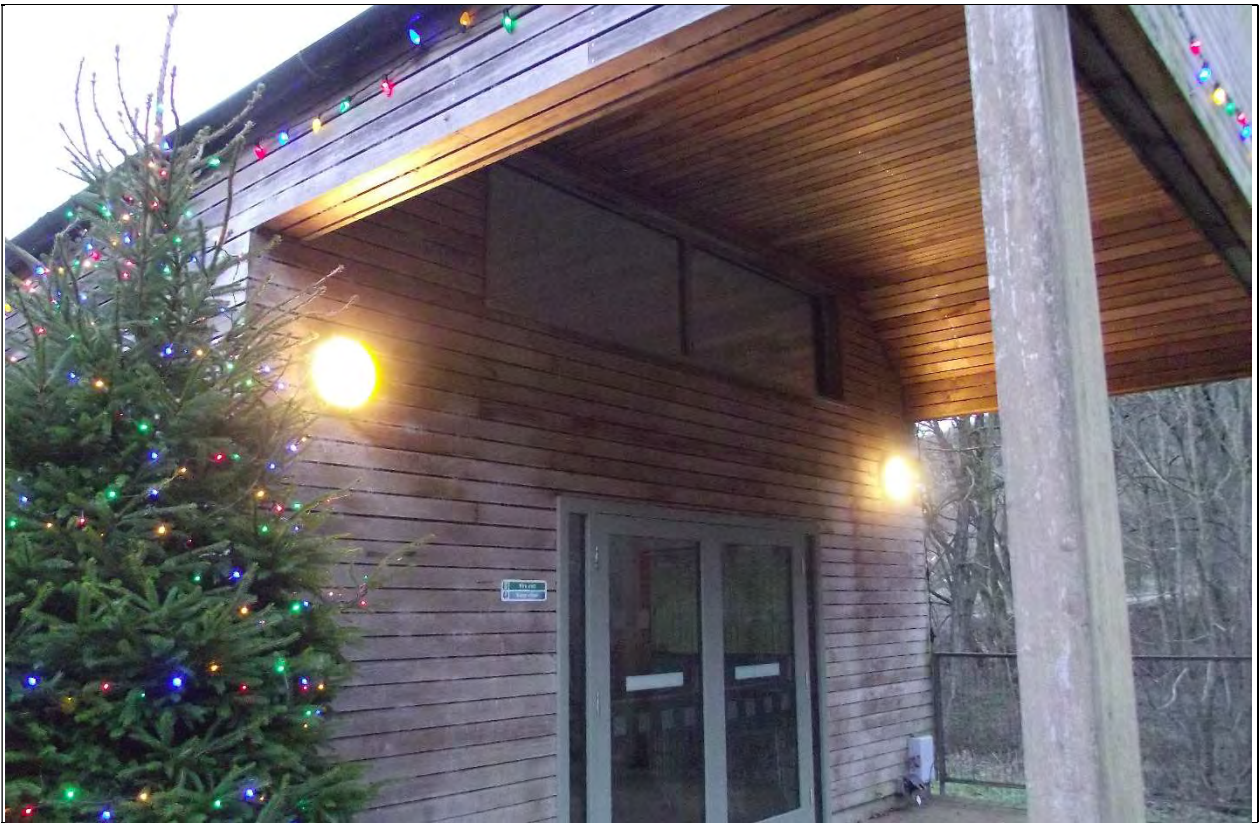
Fittings Y&Z-Locations under canopy of building within the courtyard
