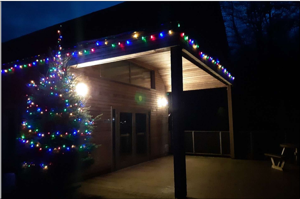
Fittings Y&Z-Locations under canopy of building within the courtyard at night
