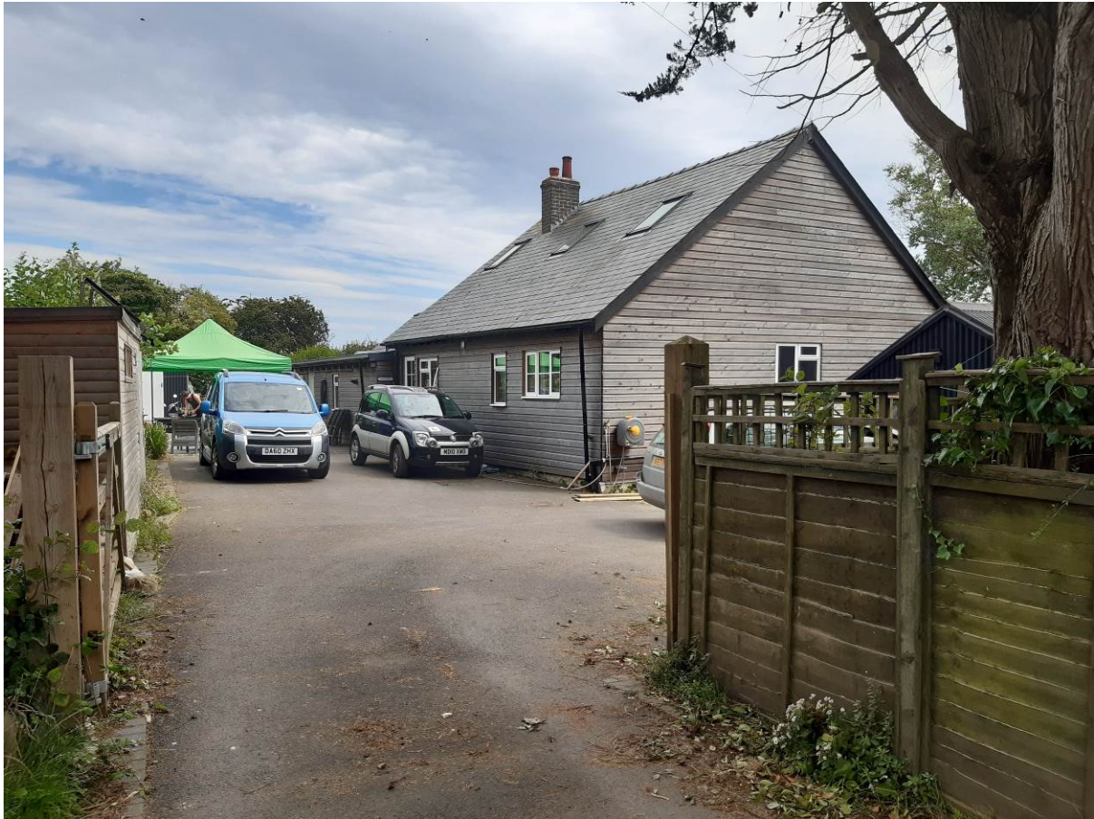
View from entrance to property with position of proposed extension beyond parked vehicles, along the rear boundary
