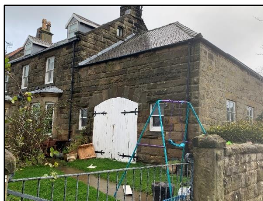
Photo 2: South-west aspect aspect of the building.
