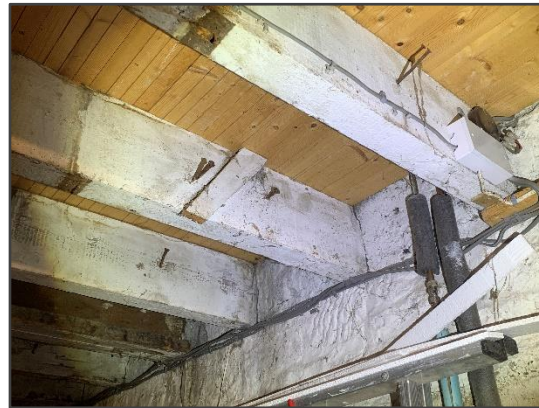
Photo 6: Ground floor boarded ceiling with timber frames.
