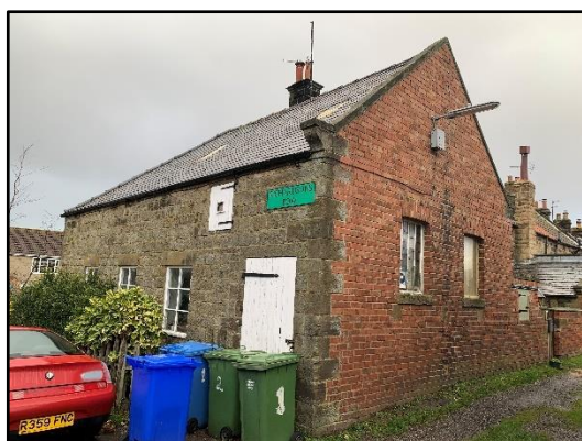
Photo 1: South-east aspect of the building.
