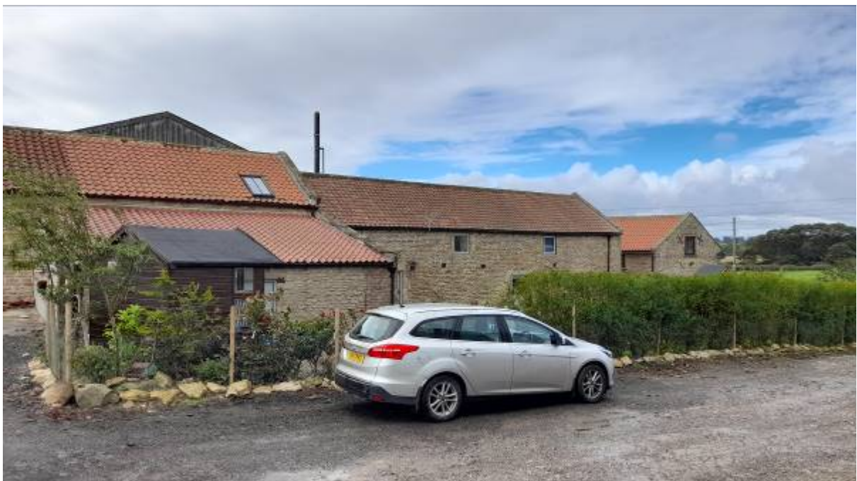
Rear Elevation of Existing Annexe
