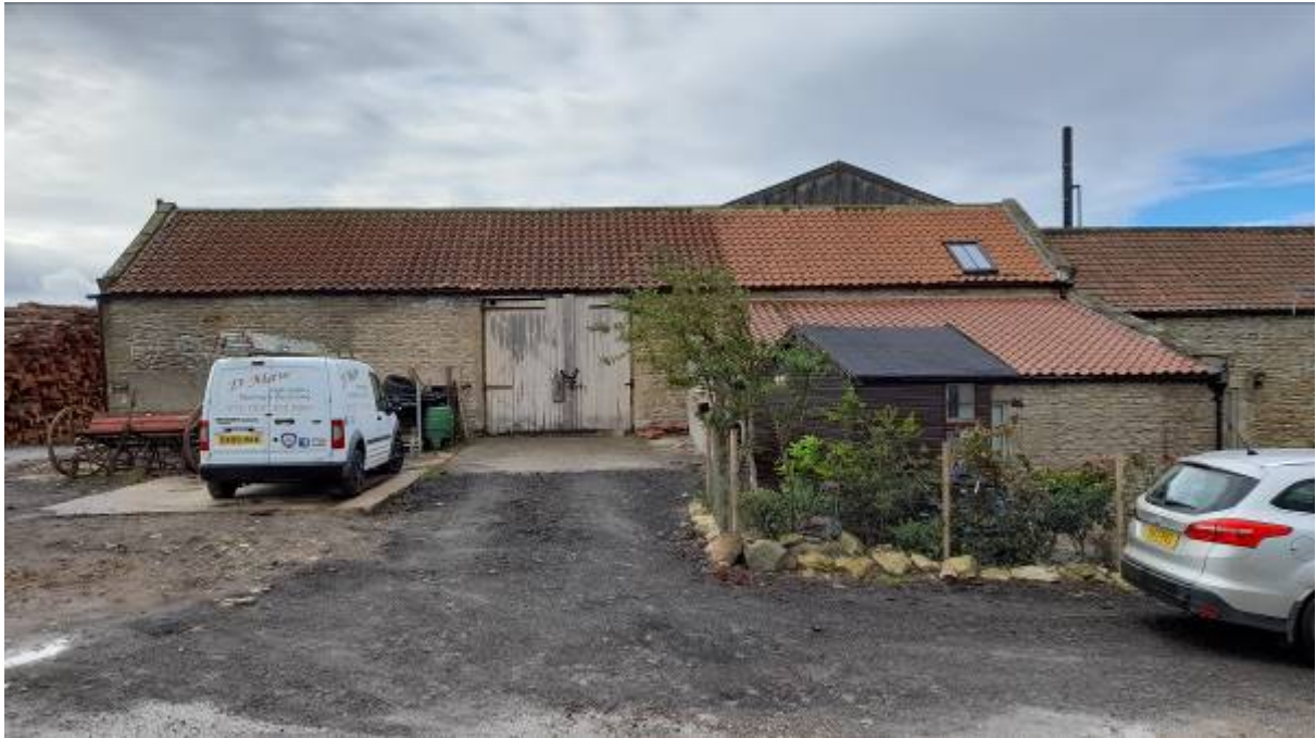
Rear Elevation of Existing Annexe and attached Barn
