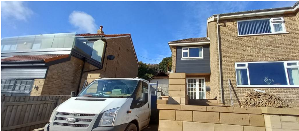
This shows the front elevation of 22 Egton Road, and the partial front elevation of 24 Egton Road which is characterised by a glazed balcony.
