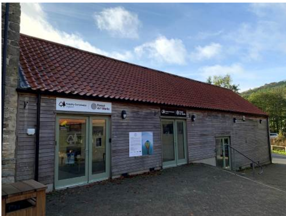
Photograph showing existing external lighting within the Courtyard
