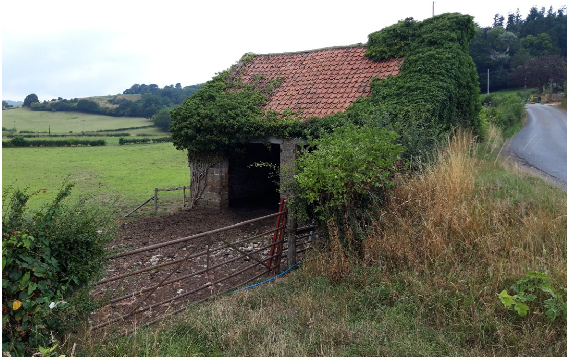
This photo shows the front of the building as existing.
