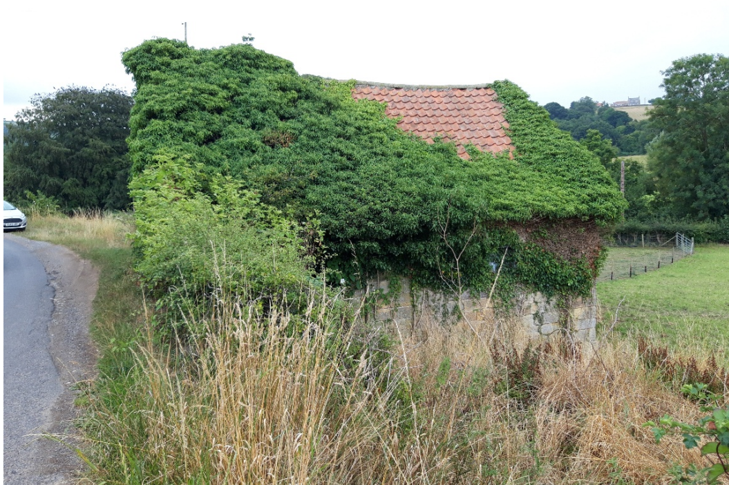
This photo shows the rear of the building as existing.
