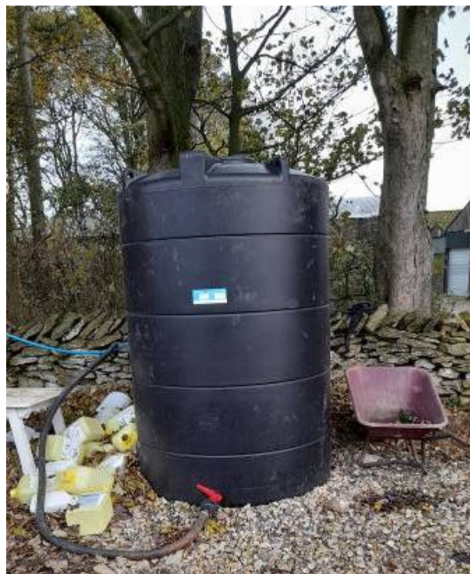
Example of water storage vessel (3000 litres) to be used on all four corners of proposed building
