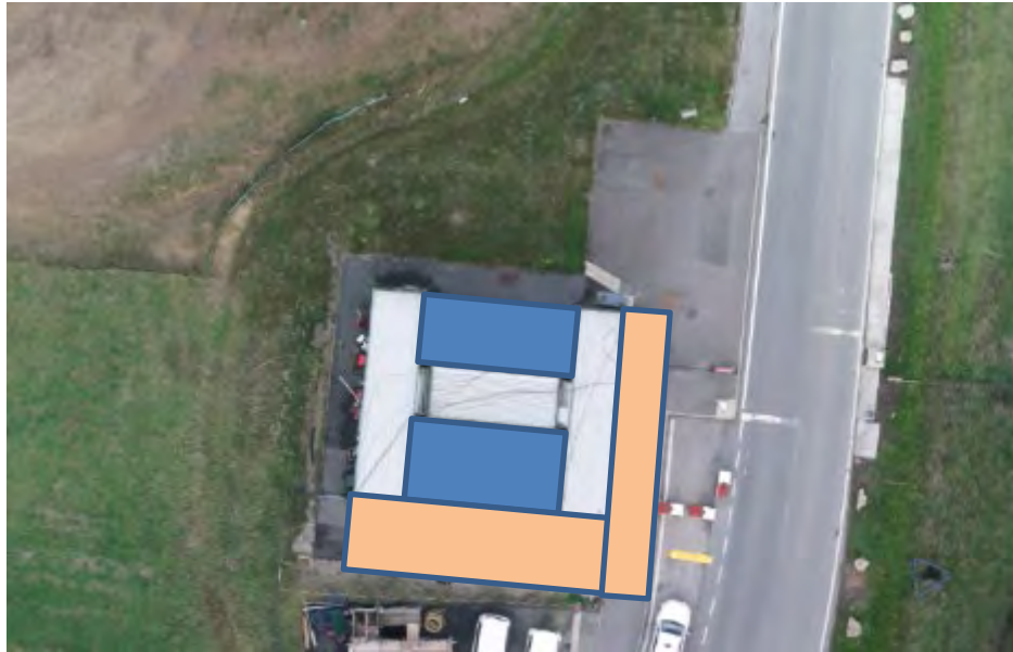
Figure 2; Security Gatehouse building
