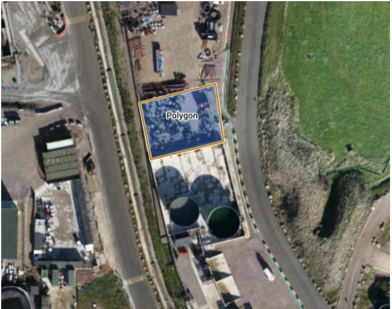
Figure 15; Process water tank relocation
