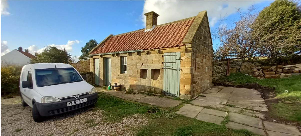
This photograph shows the outbuilding to the north of the main dwelling.
